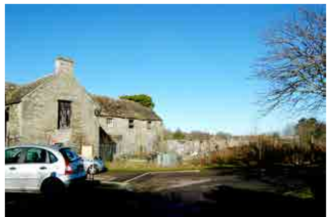
View of the existing derelict Millbank buildings
