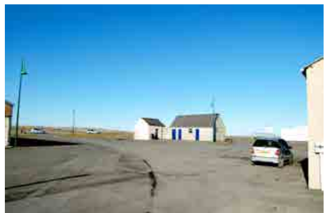
Existing buildings on promontory
