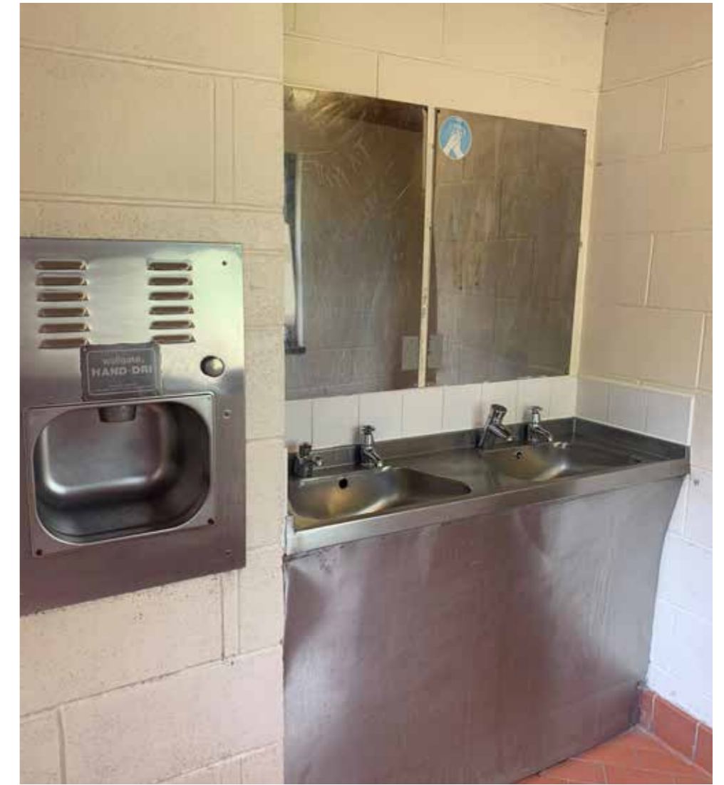
Existing Female Toilets
