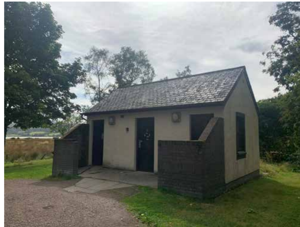
View of existing toilets
