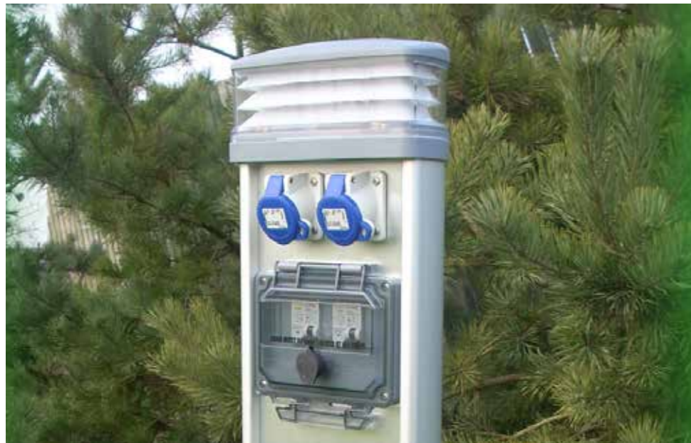
RMCS - Detail of Electrical Service Pedestal
