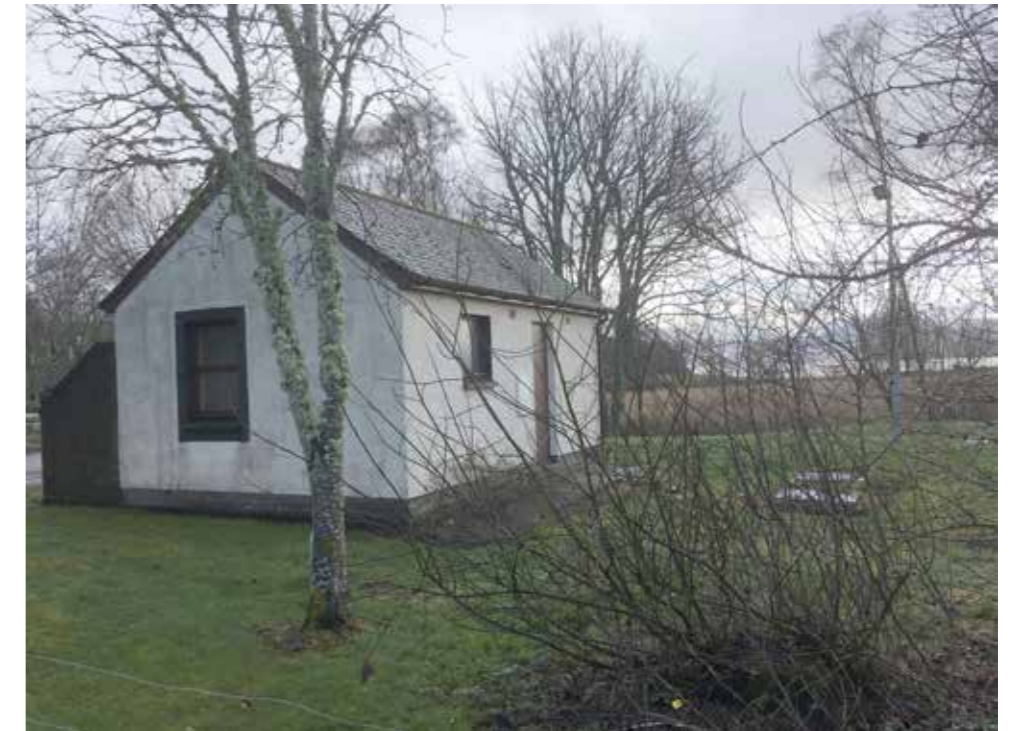
Existing WC structure with septic tank visible to right
