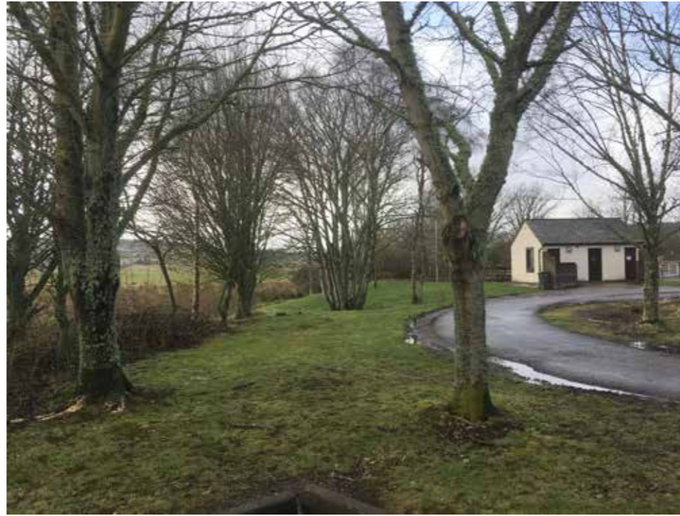
Existing WC structure to right - to be refurbished as required
