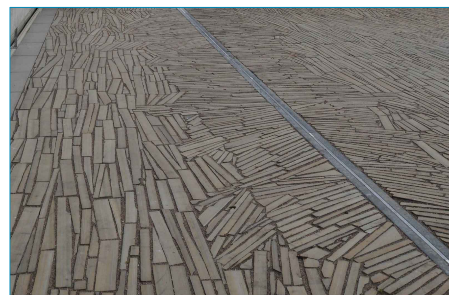
'Pocket Park' area gives views over the riverside and includes seating, paved areas and planters. The paving design combines multi-toned porphyry paving (above) and a feature paving area of Caithness flagstone laid on edge to give a 'wave pattern'. This paving could be interspersed with shoals of fish set into the paving as an element of artwork.
