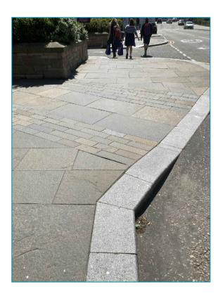
Caithness flagstone will be lifted and replaced or reused as appropriate. As the flagstone is local to Wick, the paving not only provide a sense of place but also reduces transportation costs and associated carbon footprints.
