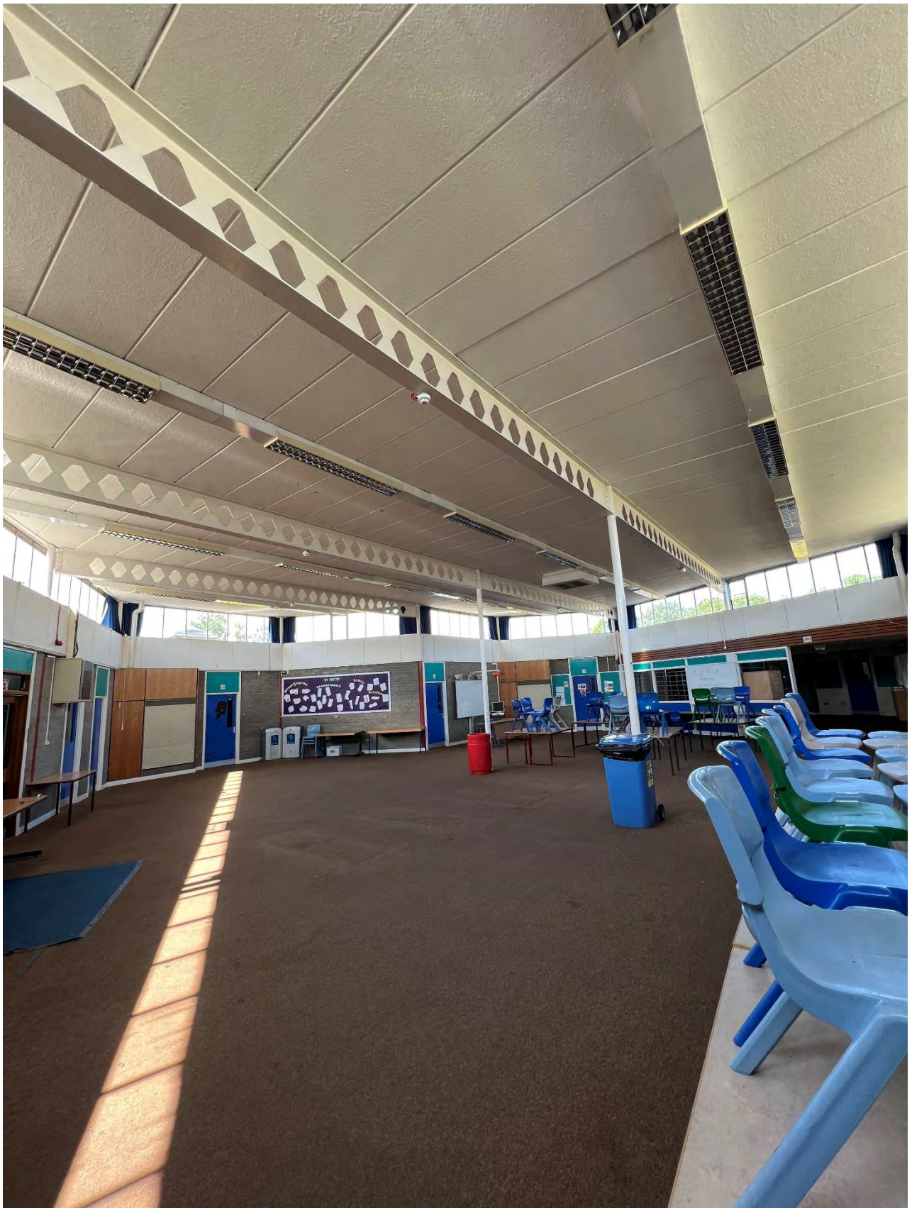
Photo N.2 Castellated beams supporting Siporex panels – flange appears to be 165mm
