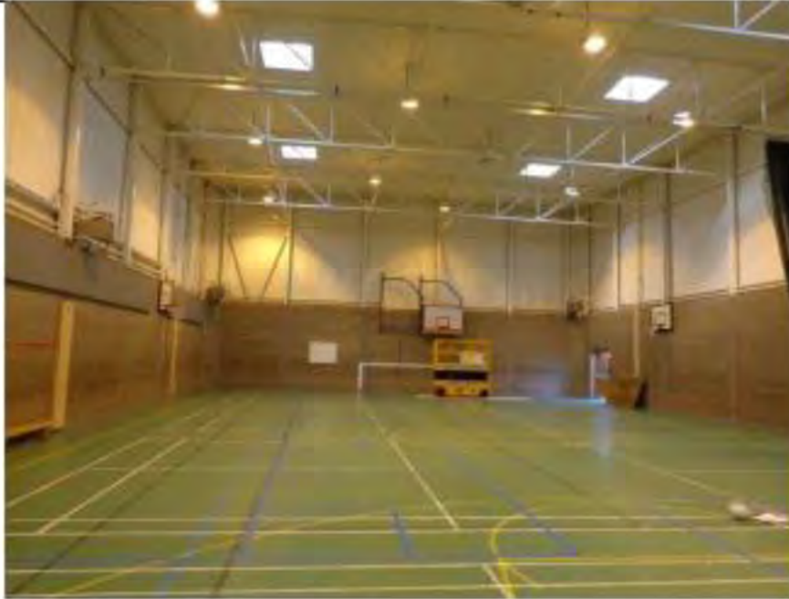
Photo No 1 – Inside Games Hall Roof & Walls
