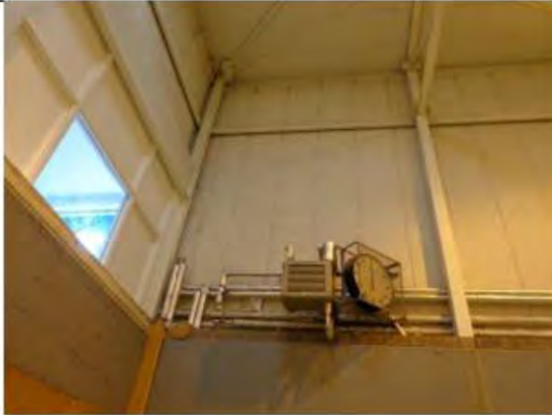
Photo No 3 – Roof & Wall Panels With Support Steelwork
