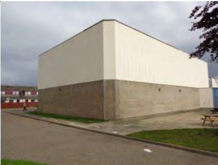
Photo No 2 – External Walls To Games Hall
