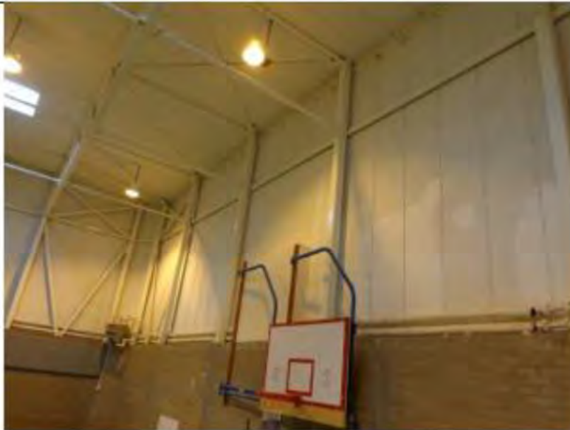
Photo No 4 – Wall Panels Above Lower Brickwork At Gable End
