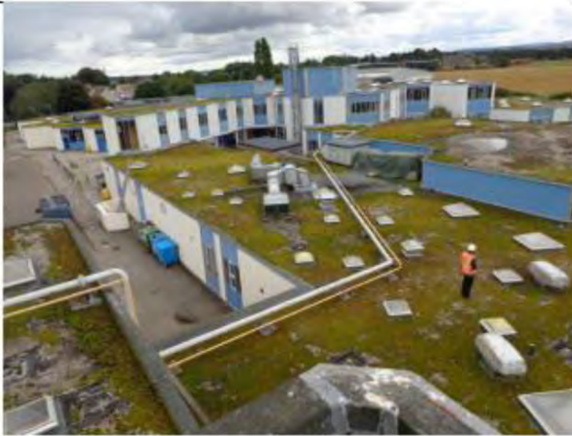
Photo No 5 – Lower Roof From Above Games Hall
