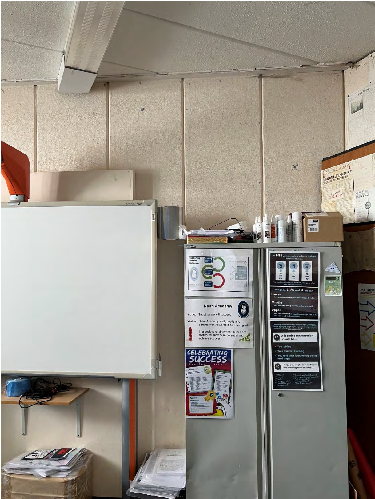
Photo N.7 Wall panels internally show no water ingress
