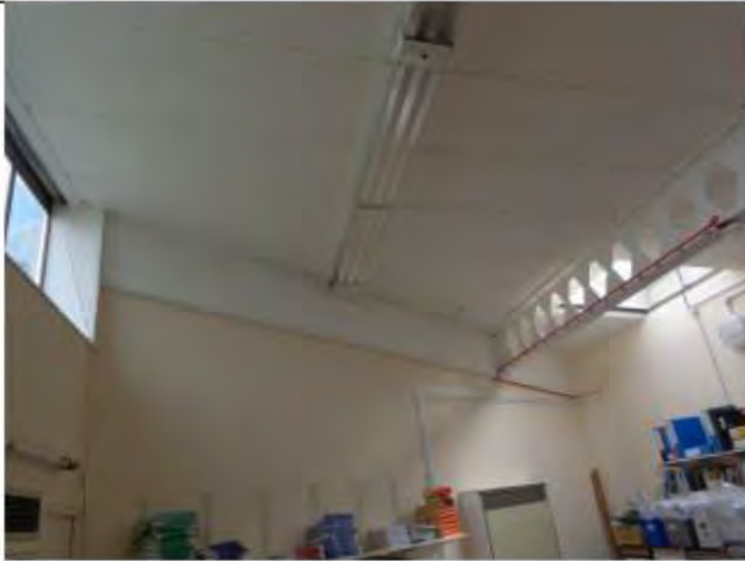
Photo No 9 – Underside Of Roof Panels Easily Checked Where No Ceiling Tiles Present
