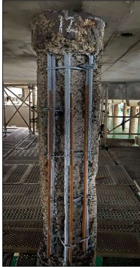
Fractured Concrete removed by hydro-dem method and reinforcing increased
