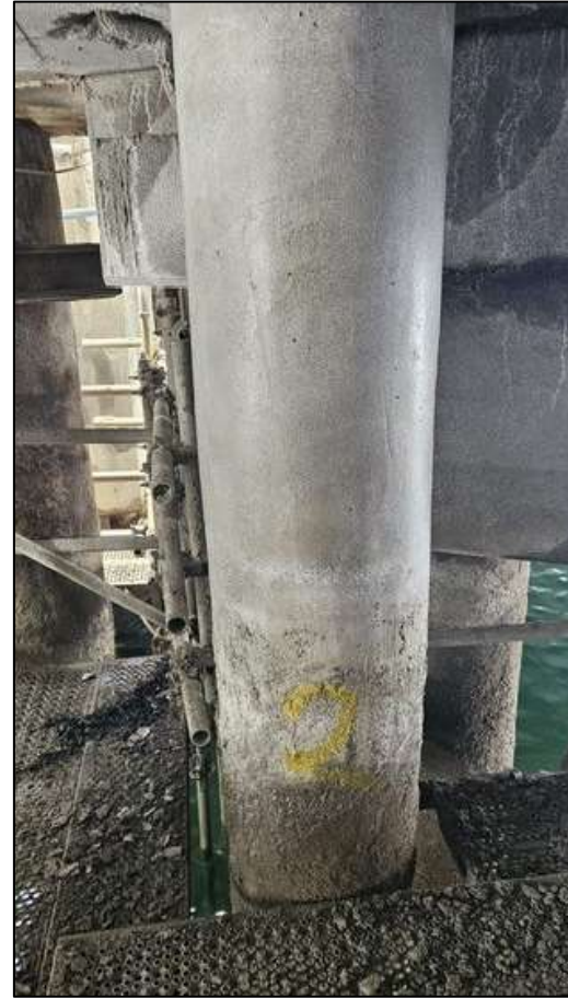
New spray on concrete formed to pile diameter.
