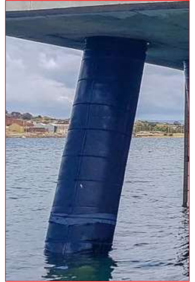
Denso wrapping applied to further protect the repair.
