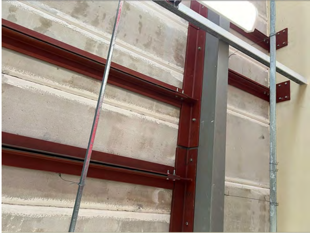
Photograph 4 – Admin Area roof light remedial supports
