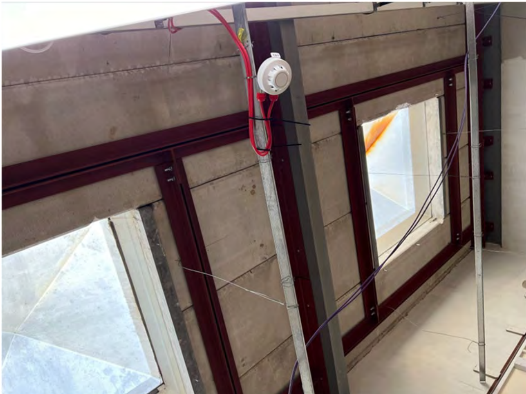
Photograph 5 – Admin Area roof light remedial supports
