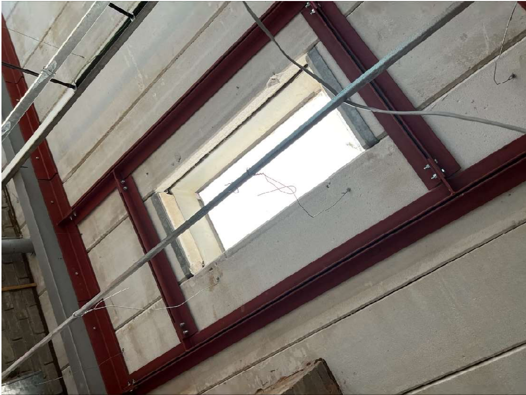
Photograph 2 – Admin Area roof light remedial supports
