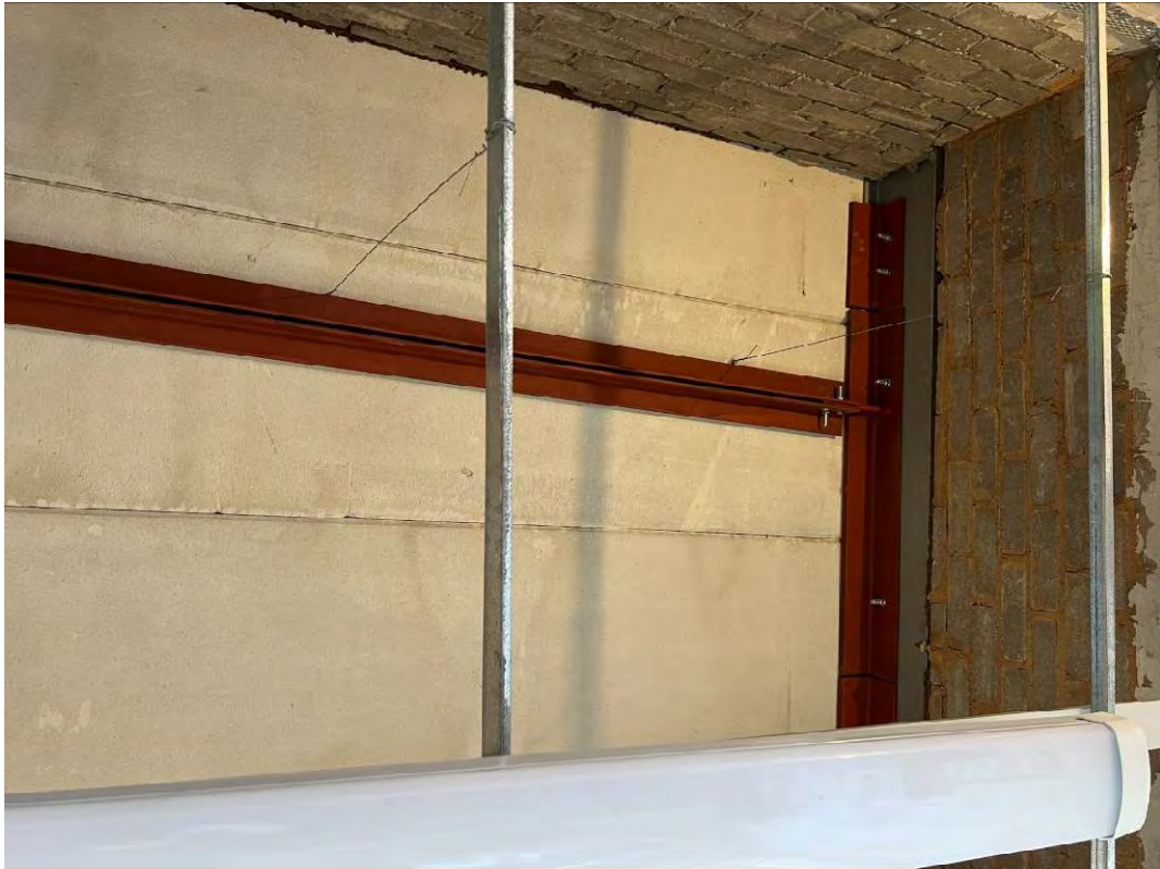
Photograph 6 – Admin Area roof light remedial supports
