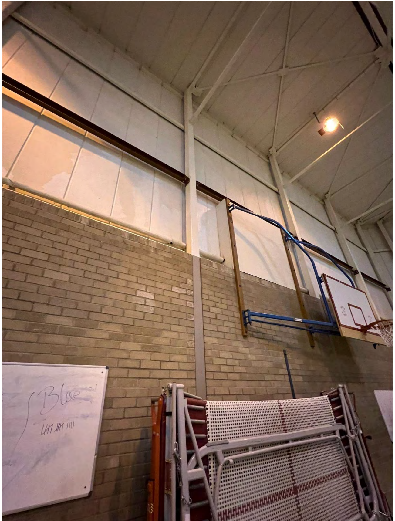
Photograph 3 – Gym Hall support beam connection details
