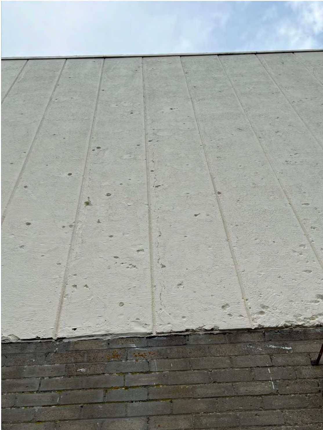
Photograph 1 – Gym Hall external panels post painting
