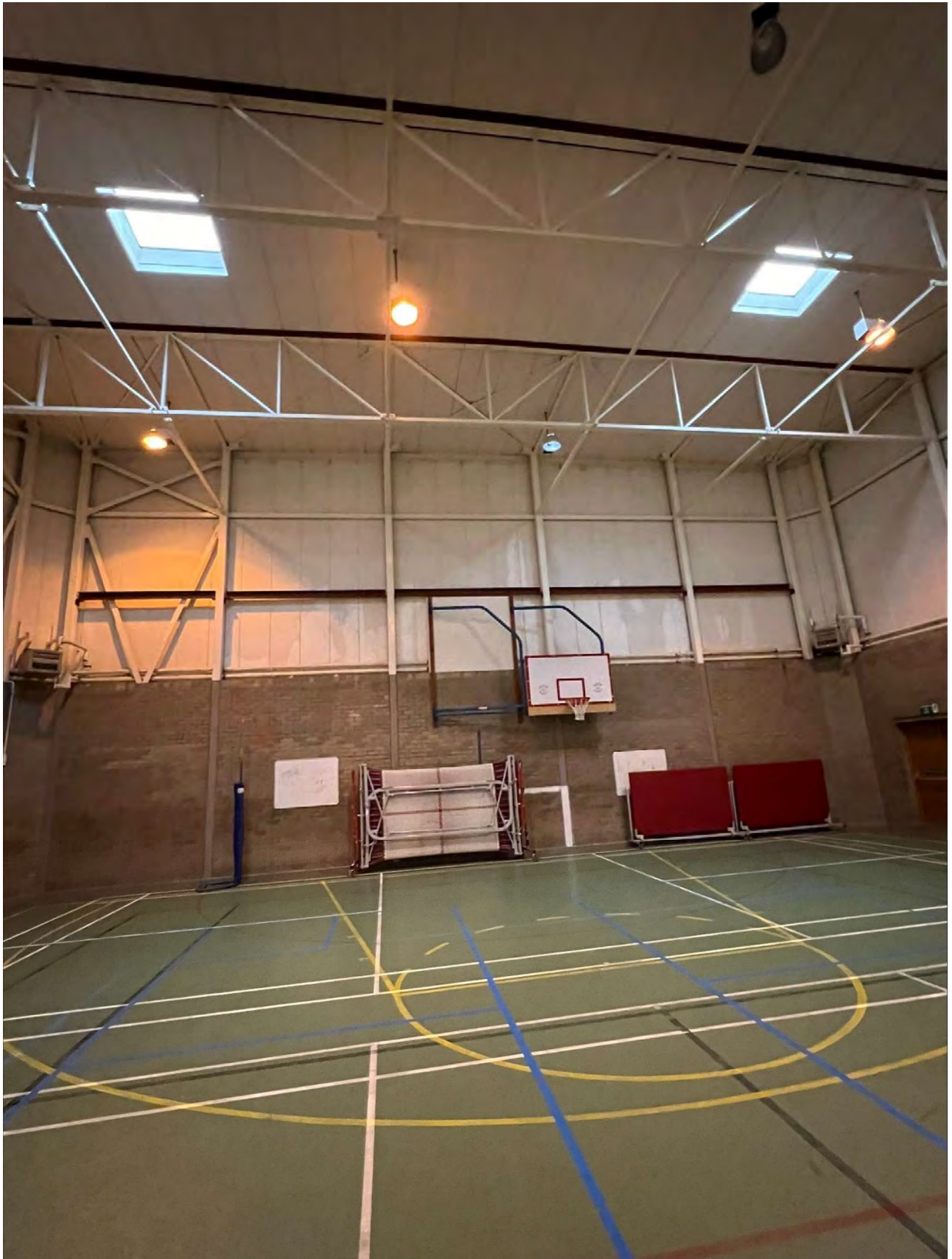
Photograph 2 – Gym hall internal mid height horizontal supports for external panels
