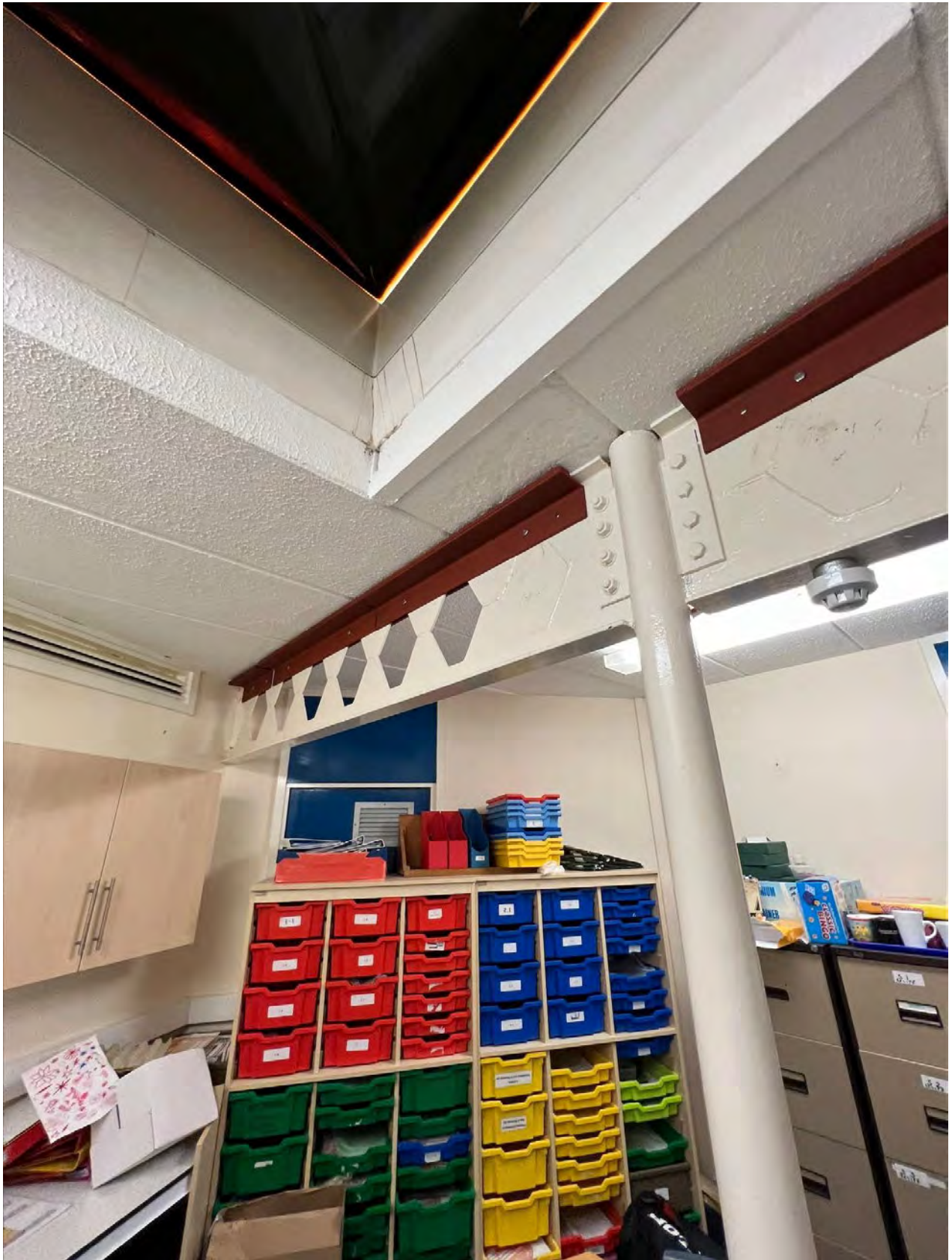
Photograph 9 – Art Dept Castellated beam extended bearing
