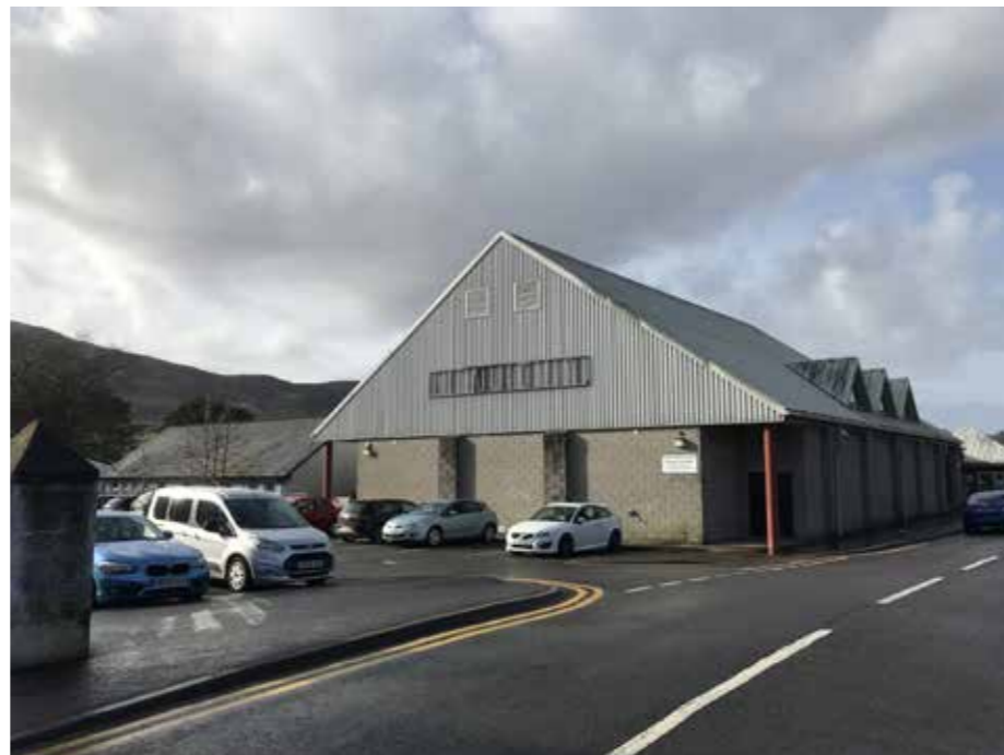
West elevation and car park
