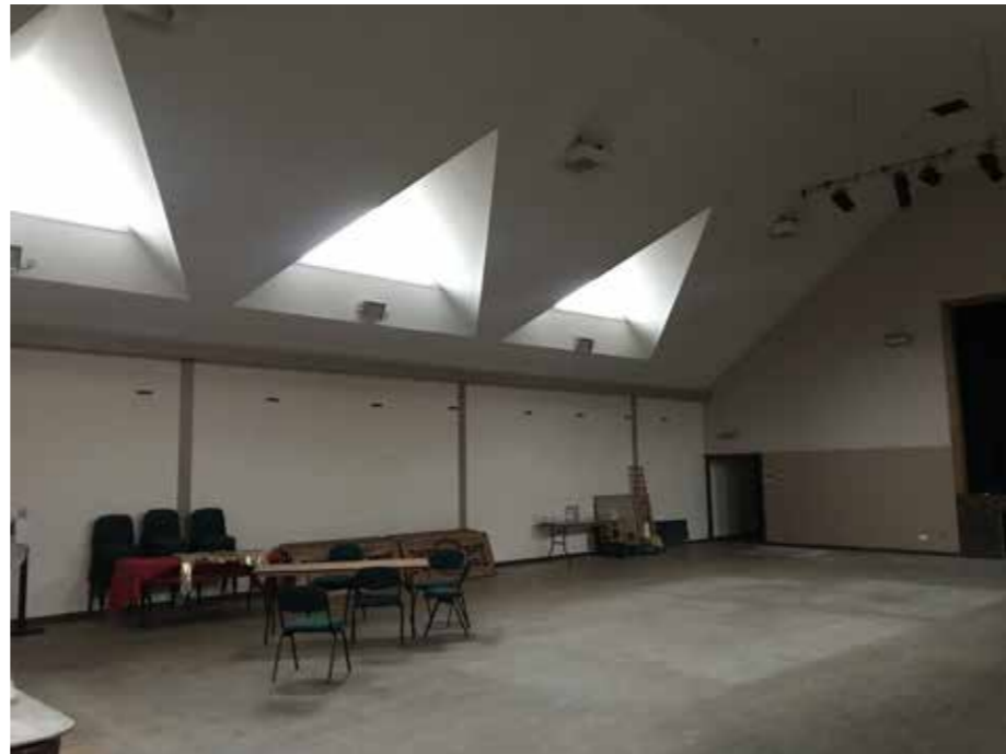
Internal north elevation
