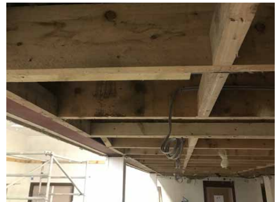
Exposed ceiling structure.
