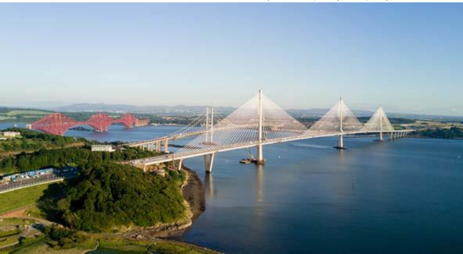
Figure 17: Queensferry Crossing (Cable Stayed Bridge)
