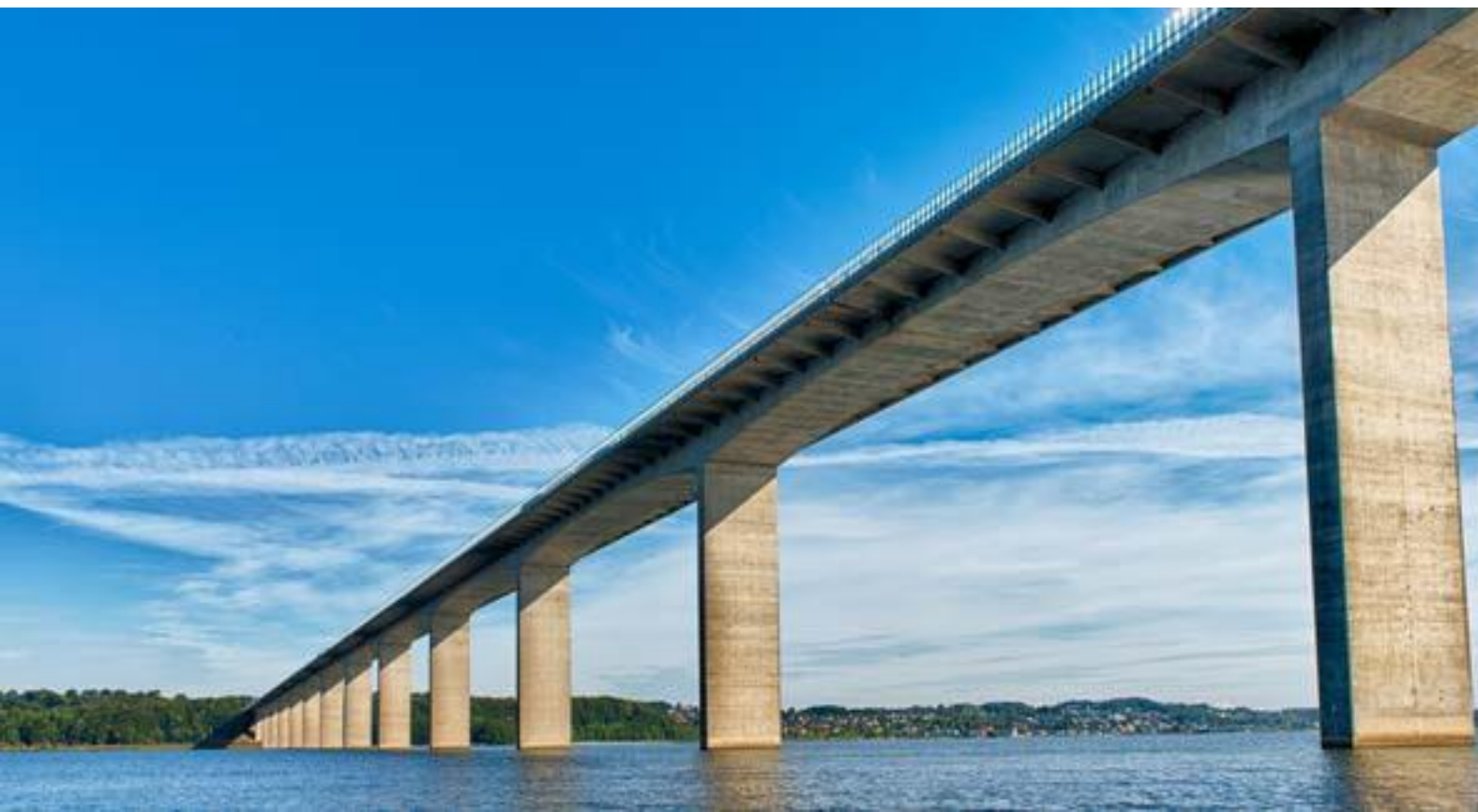
Figure 21: Vejle Bridge (Cantilever Bridge)
