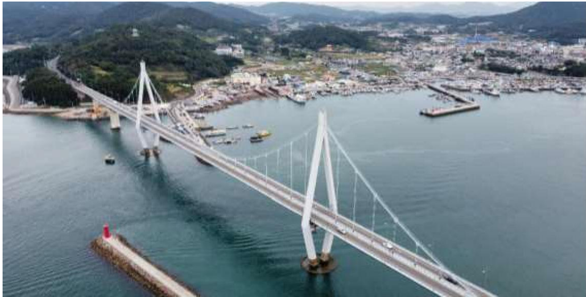
Figure 3-19: Sorok Suspension Bridge (South Korea)
