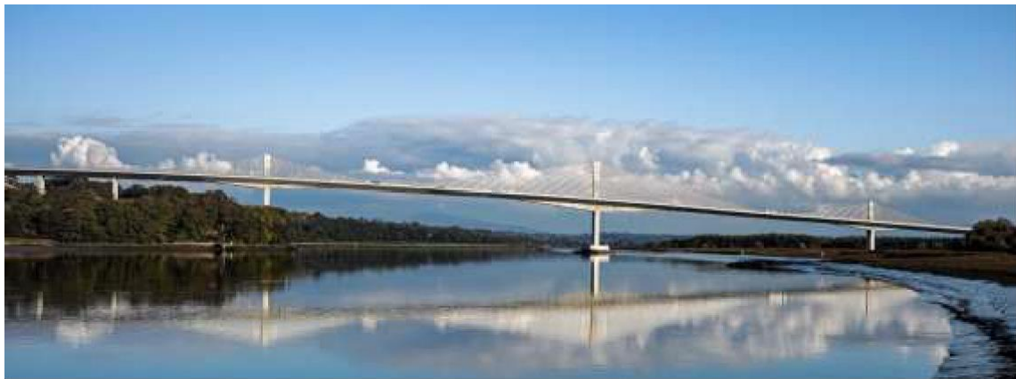
Figure 3-15: Rose Fitzgerald Kennedy Bridge (Ireland)
