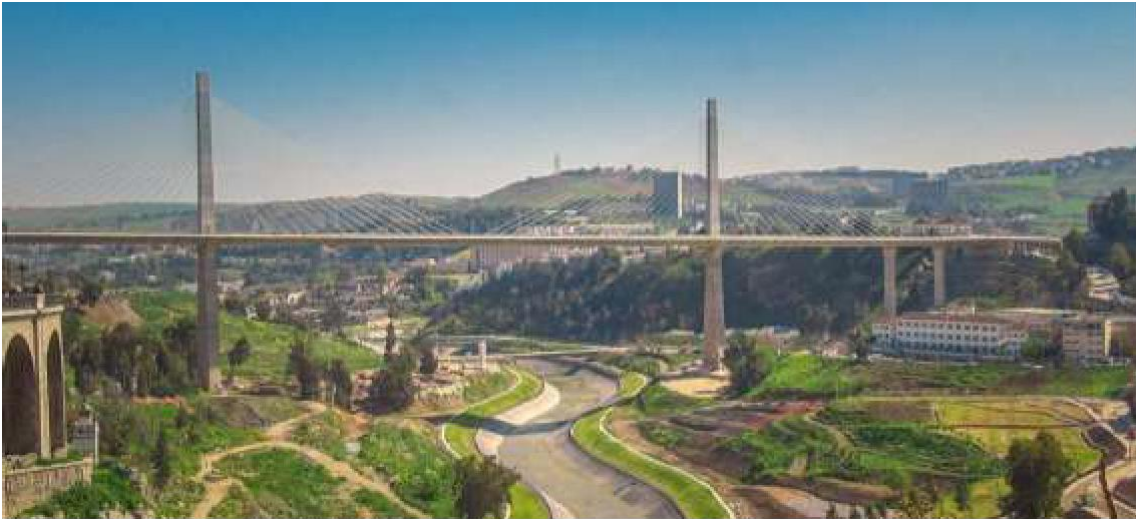
Figure 3-17: Salah Bey Viaduct (Constantine Bridge) in Algeria
