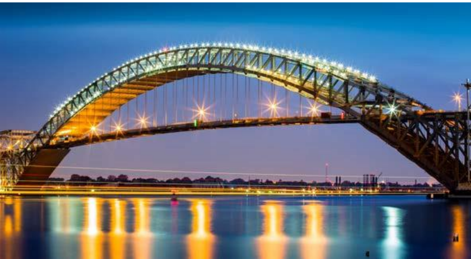
Figure 19: Bayonne Bridge (Tied Arch Bridge)
