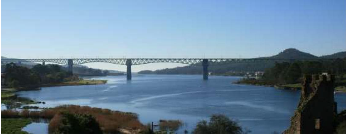
Figure 3-6: Ulla Viaduct (Spain)
