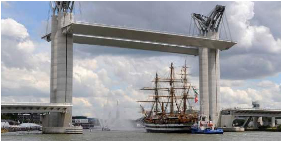
Figure 3-23: Gustave Flaubert Bridge (France)
