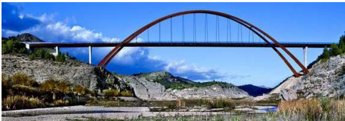
Figure 3-13: Vicaria Bridge, Spain
