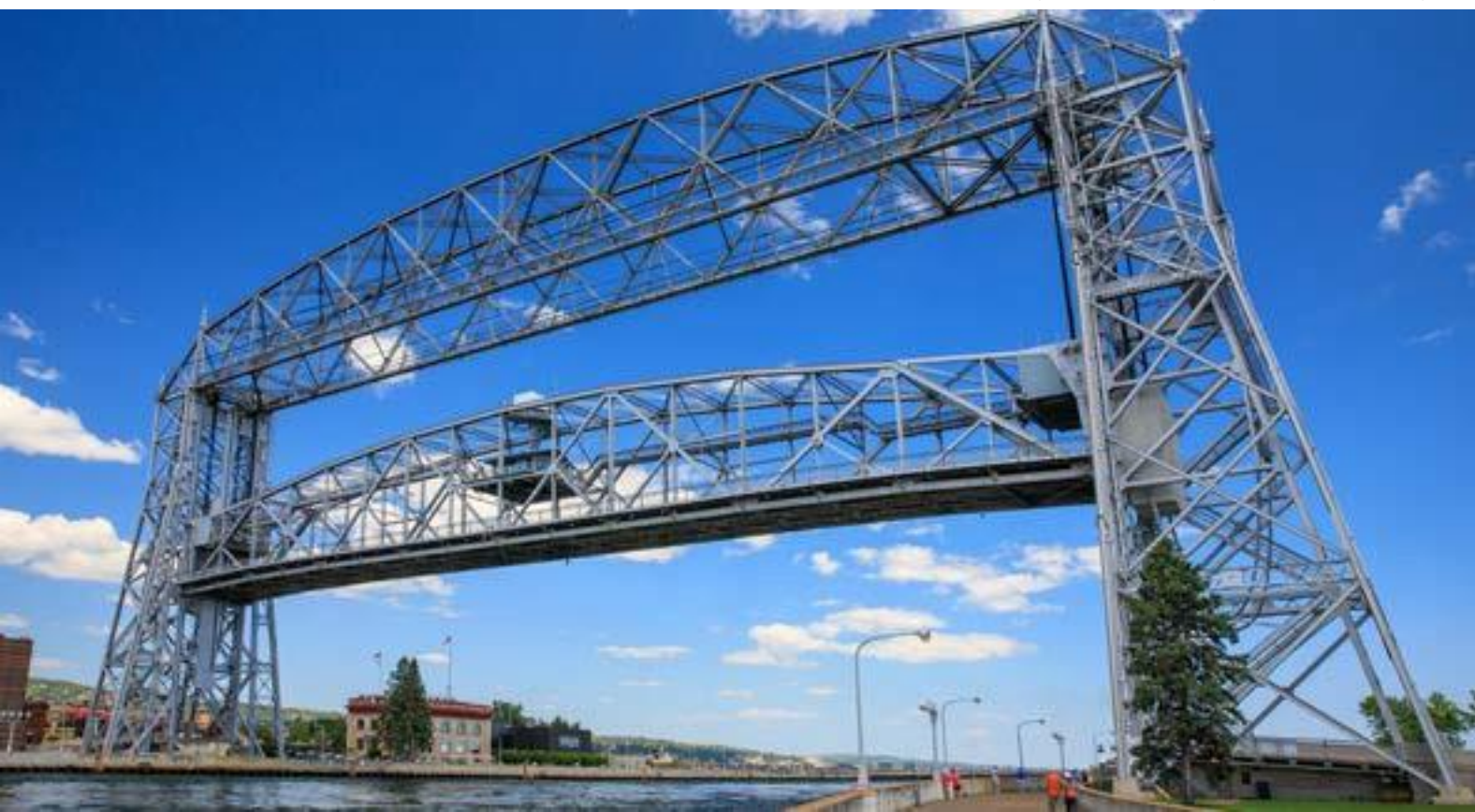
Figure 20: Aerial Lift Bridge, Duluth (Vertical Lift Bridge)
