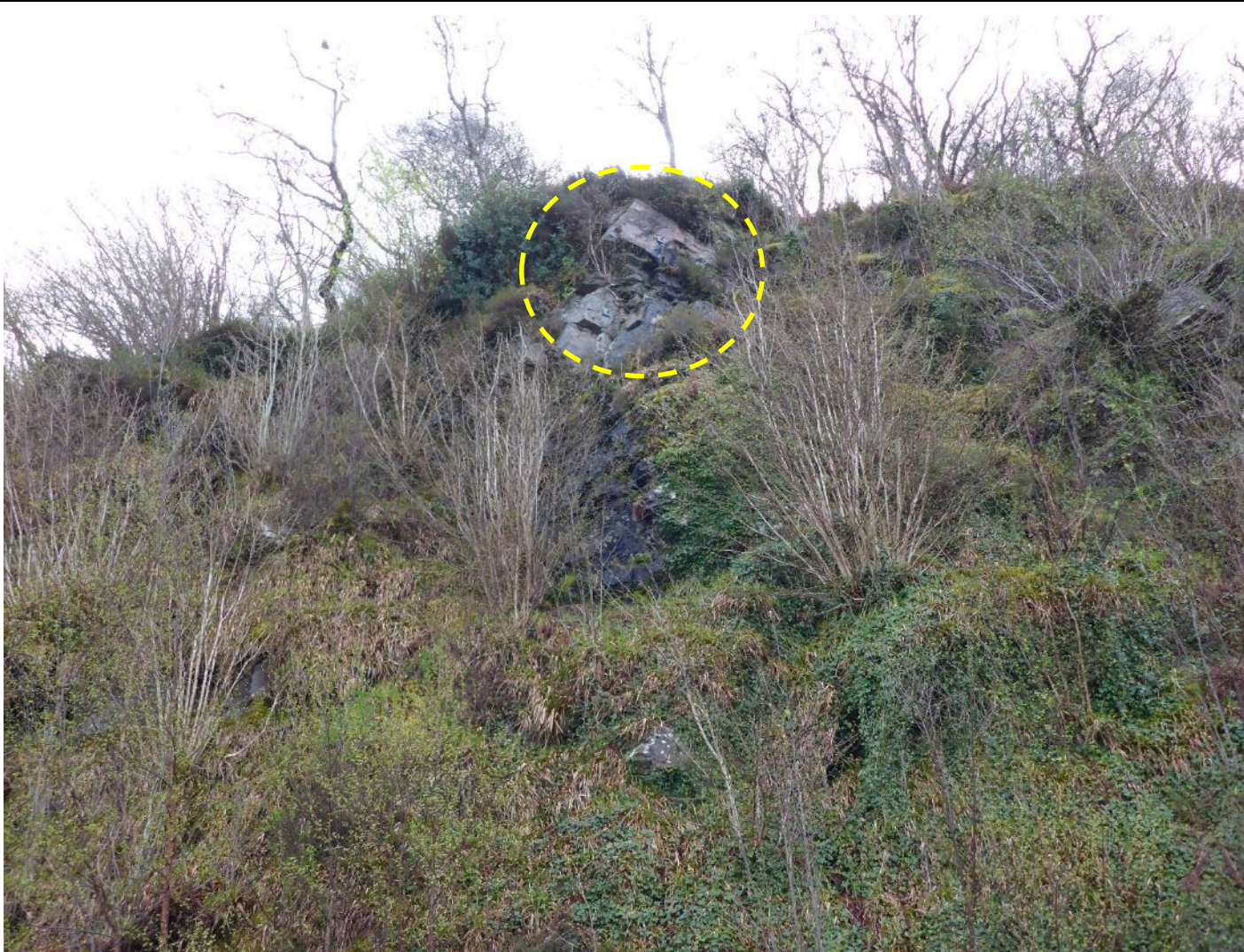
Ch. 788 – Overhanging block at crest of slope.
