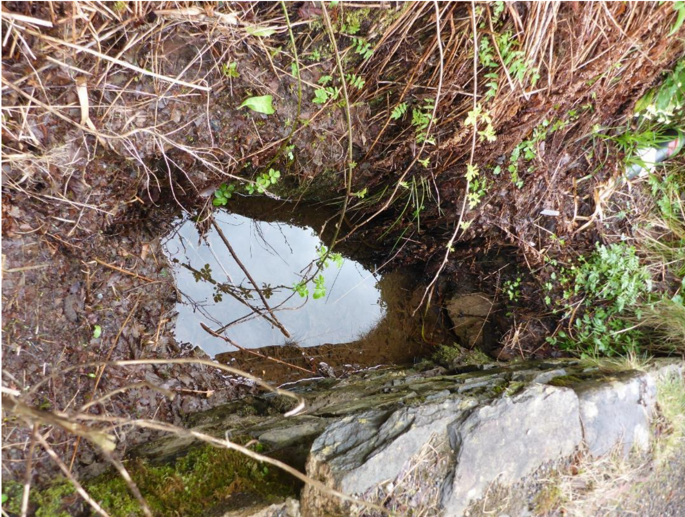
Ch. 1832 – Drainage gully blocked.
