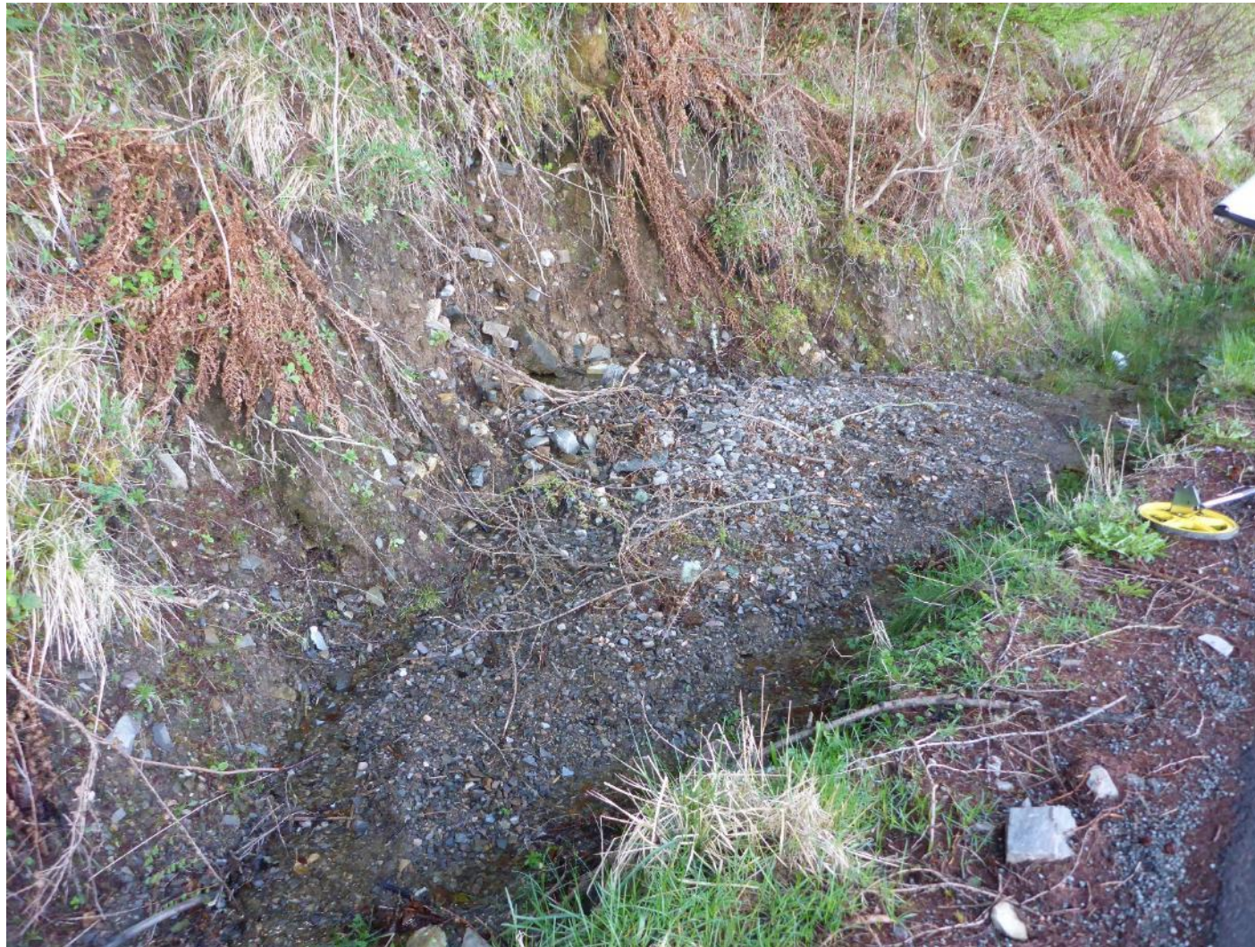
Ch. 428 – Ditch filled with small granular debris at toe of ephemeral watercourse.
