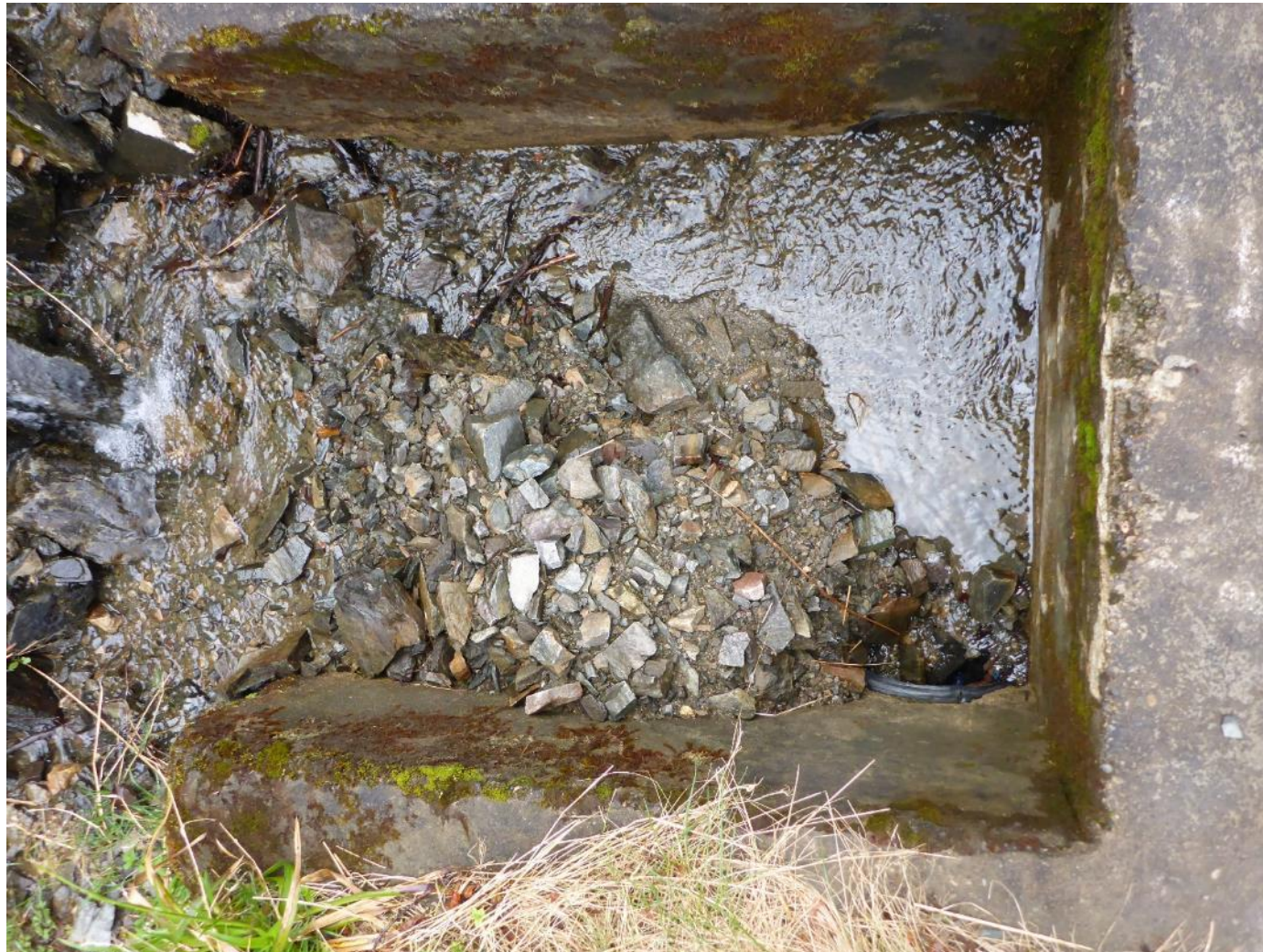
Ch. 1825 – Debris in drainage gully nearly at gully capacity.
