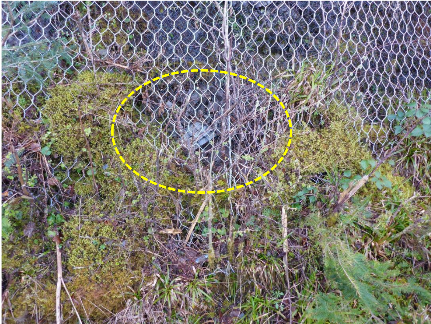
Ch. 190 – Accumulation of small blocks behind netting. (Feature circled).
