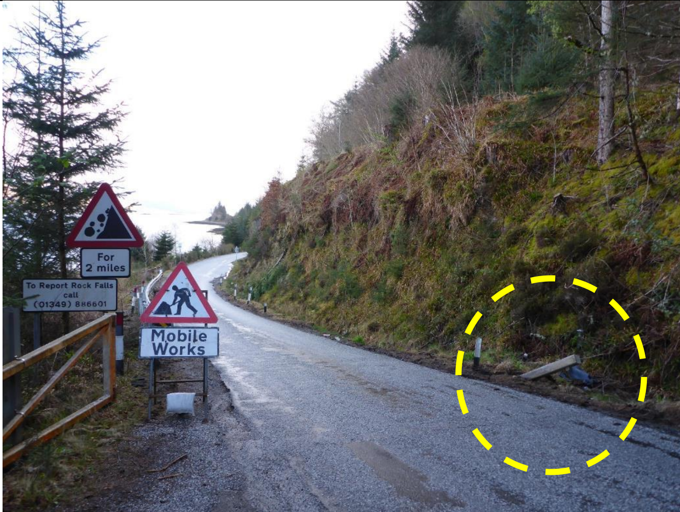
Ch. 0 – Road closure gate post has been struck and knocked over. Feature circled.
