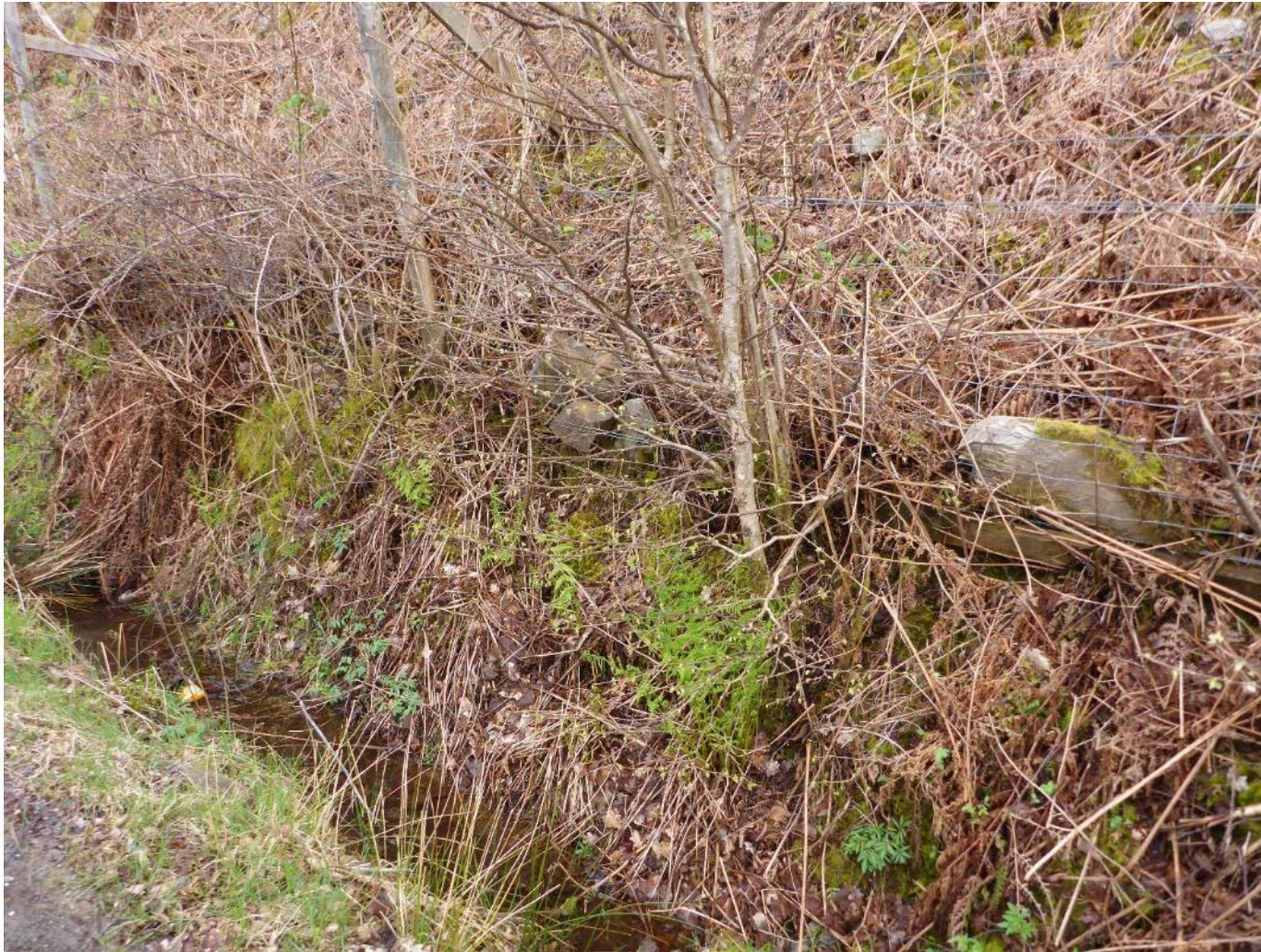
Ch. 1323 – Several small rocks accumulated at deer fence or burst through and landed in ditch.
