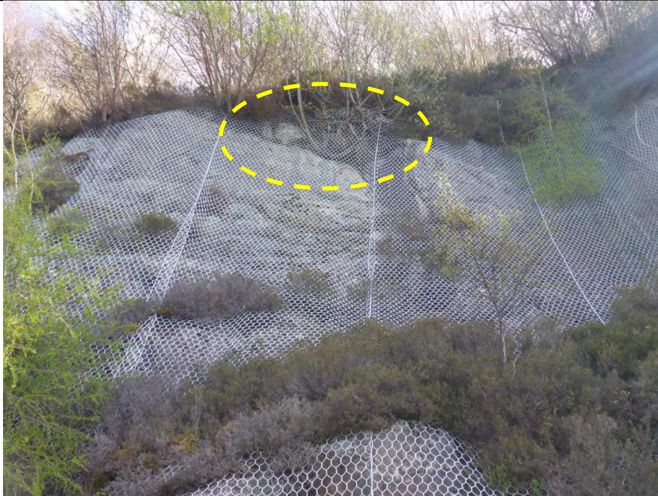
Ch. 3363 – Broken rock mass at crest. Root jacking an issue.
