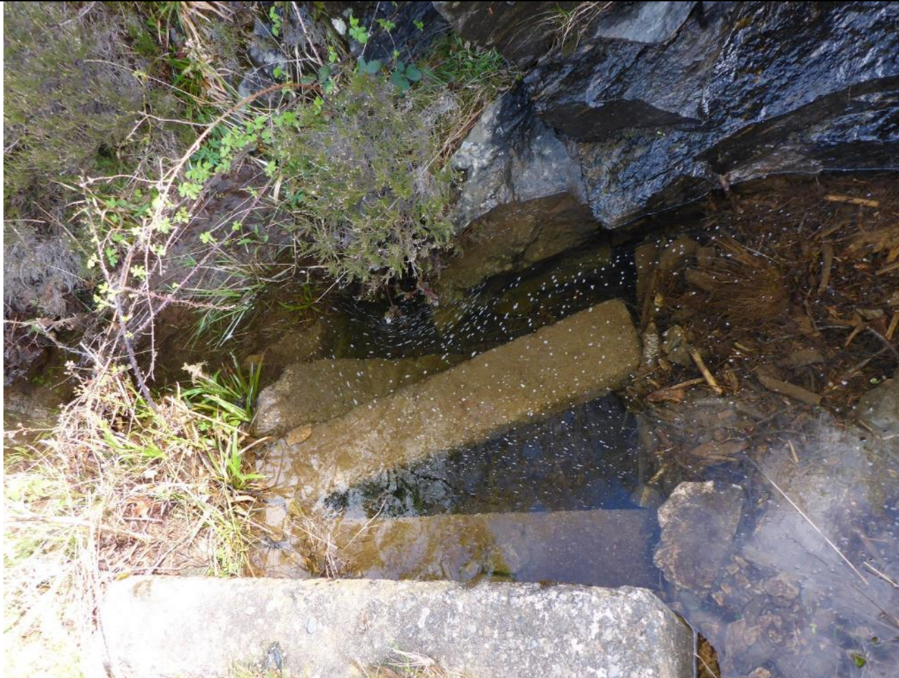
Ch. 3380 – Blocked culvert.
