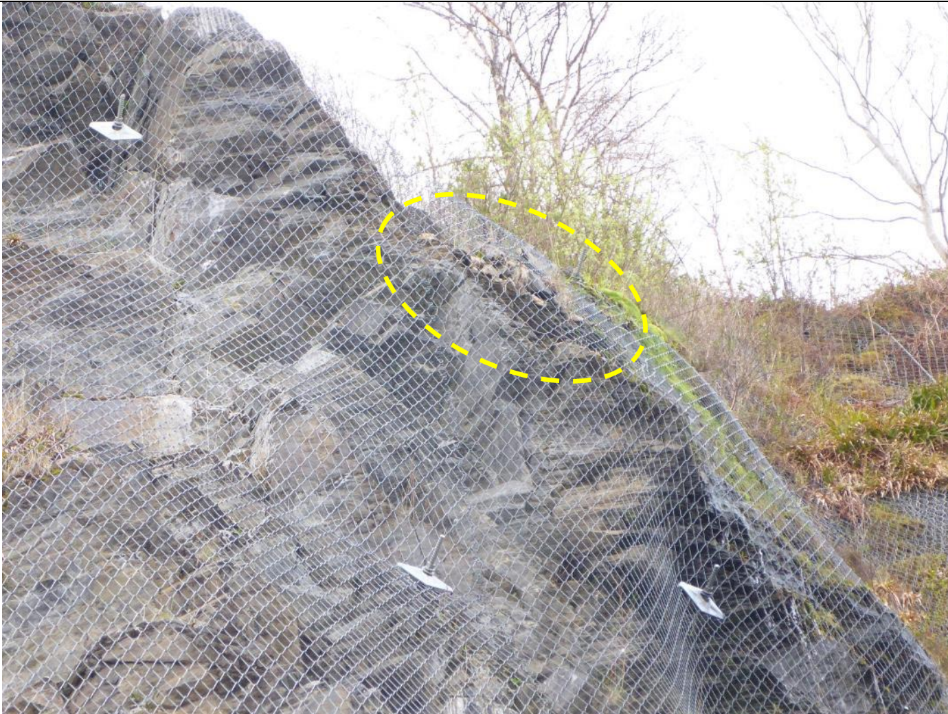
Ch. 2990 – Some loose blocks behind netting near crest of slope.
