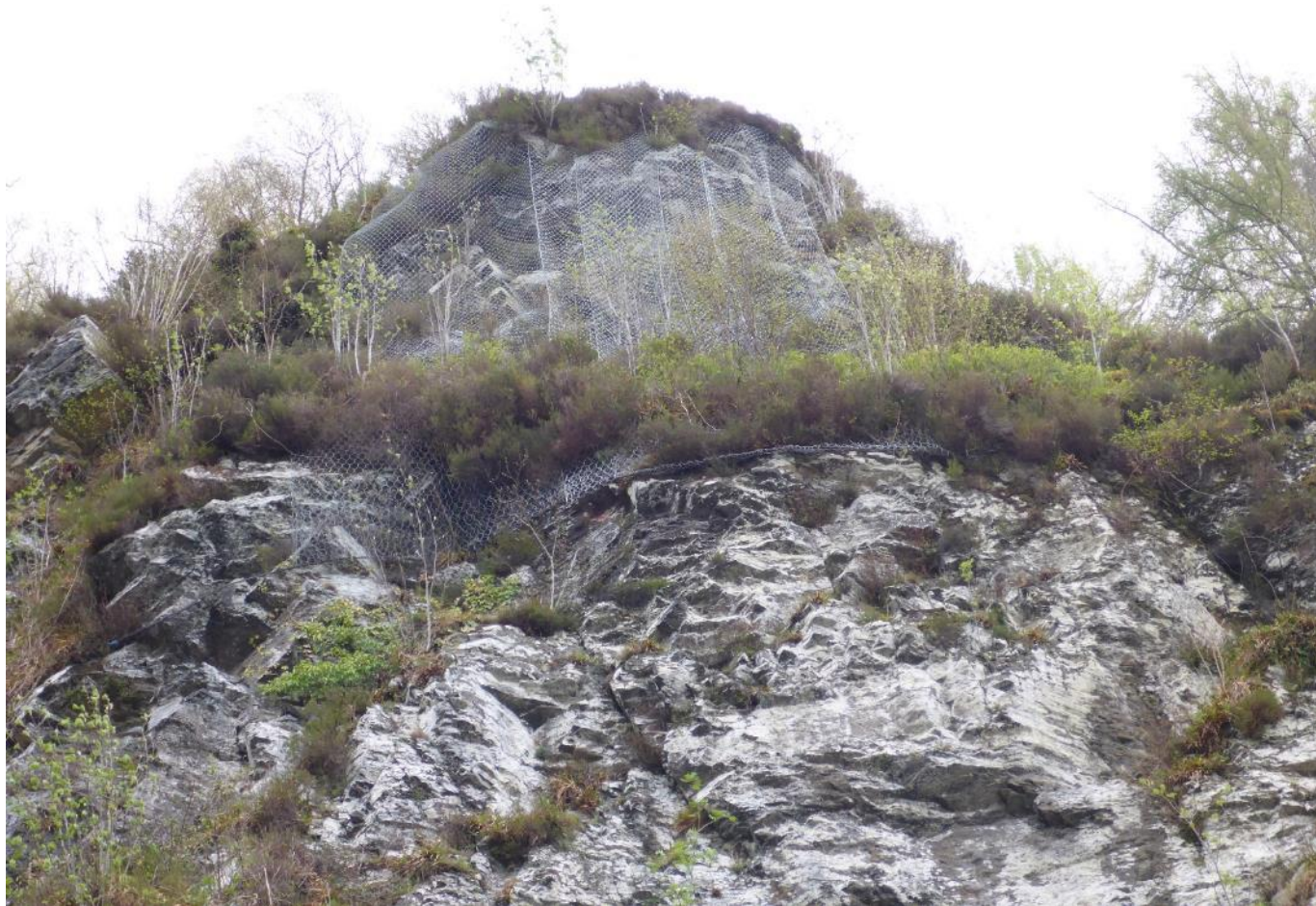
Between Ch. 1965 to 1975 – Netting noted to be gaping at sides and bottom.
