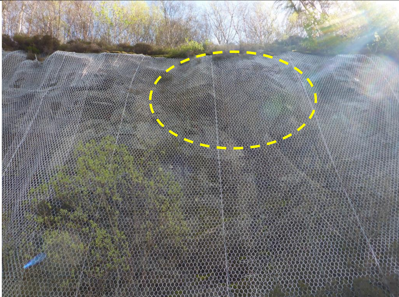
Ch. 3305 – Large wedge at crest of rock slope behind netting.
