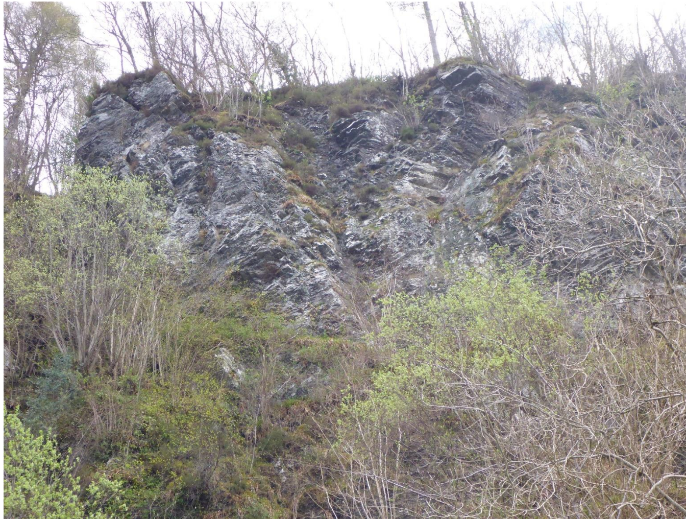
Ch. 2000 – Large scale wedge failure potential at crest of rock slope.
