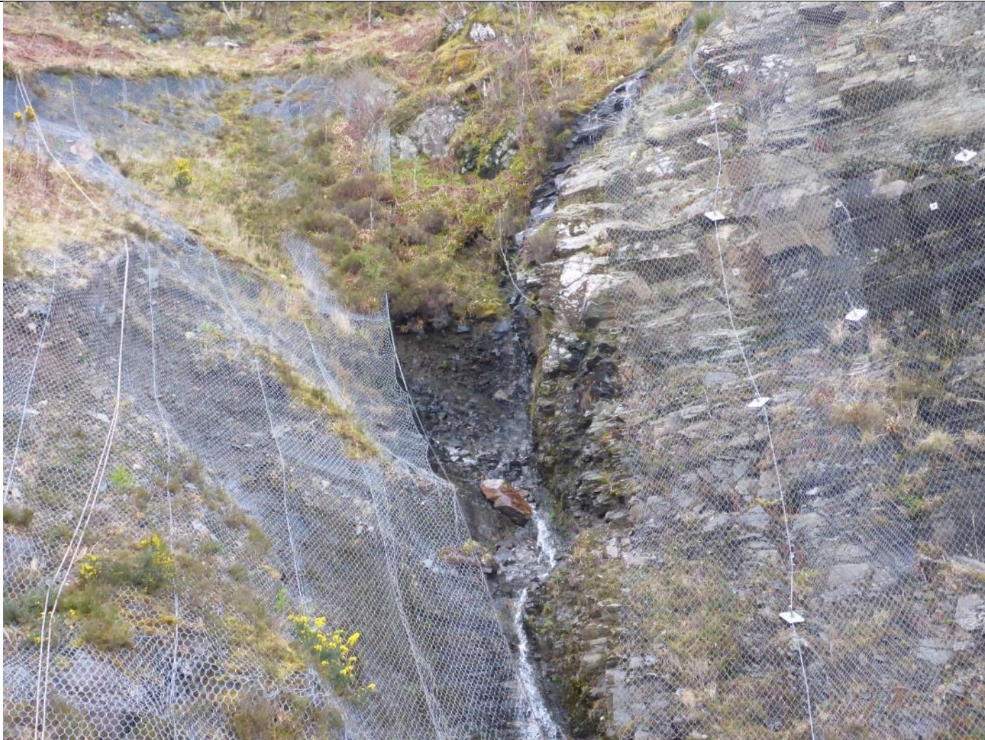
Ch. 3059 – Washout at base of waterfall and mid slope about 10m above road level.
