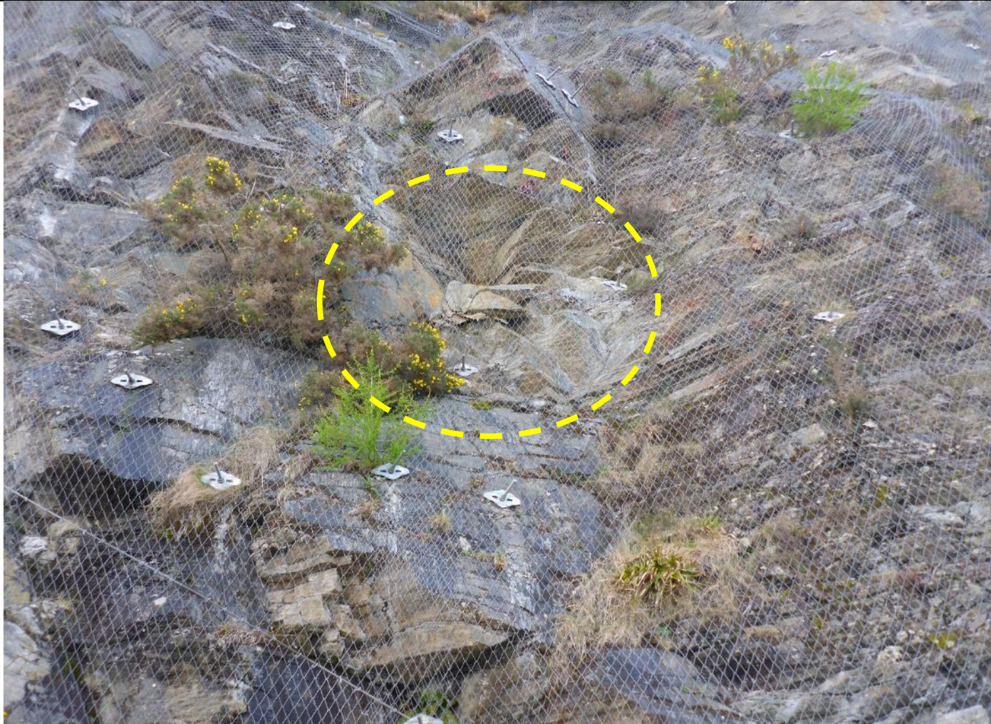
Ch. 3100 - Failure of ca. 0.25m 3 block observed 6-8m above road level and has been retained by mesh.
