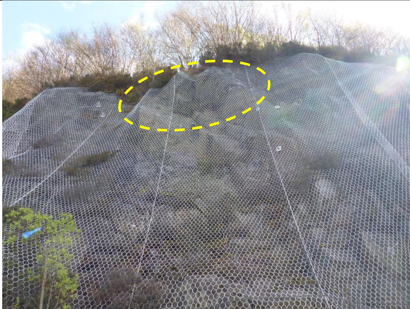
Ch. 3350 – Overhanging rock mass at crest with dilated release plane.
