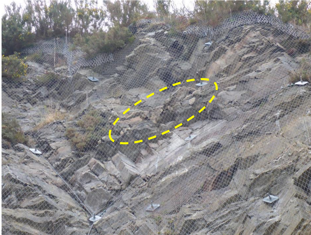
General – localised small blocks (ravelling) behind TECCO c. 15-20m upslope of buttress.
