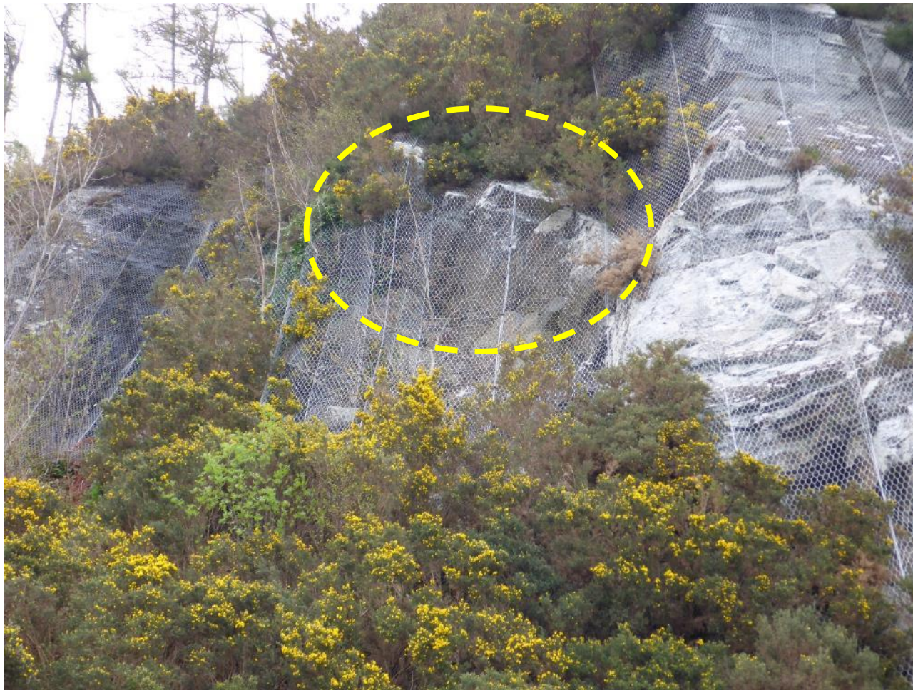
Ch. 2535 – Overhang area c. 12 to 15m above toe with gapping mesh below.
