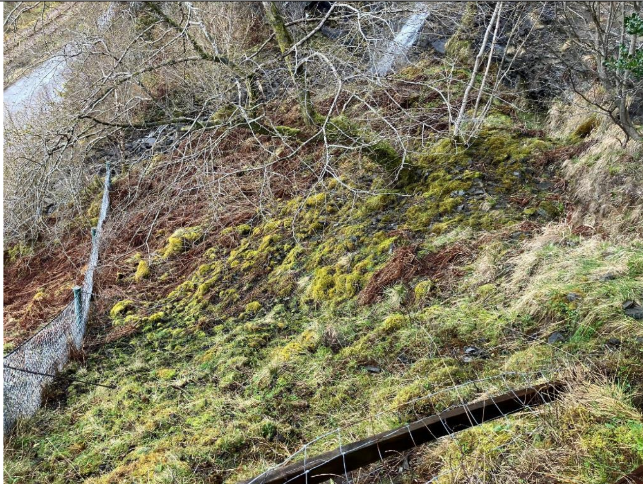
Mid-slope catch fence 1.5m high.
