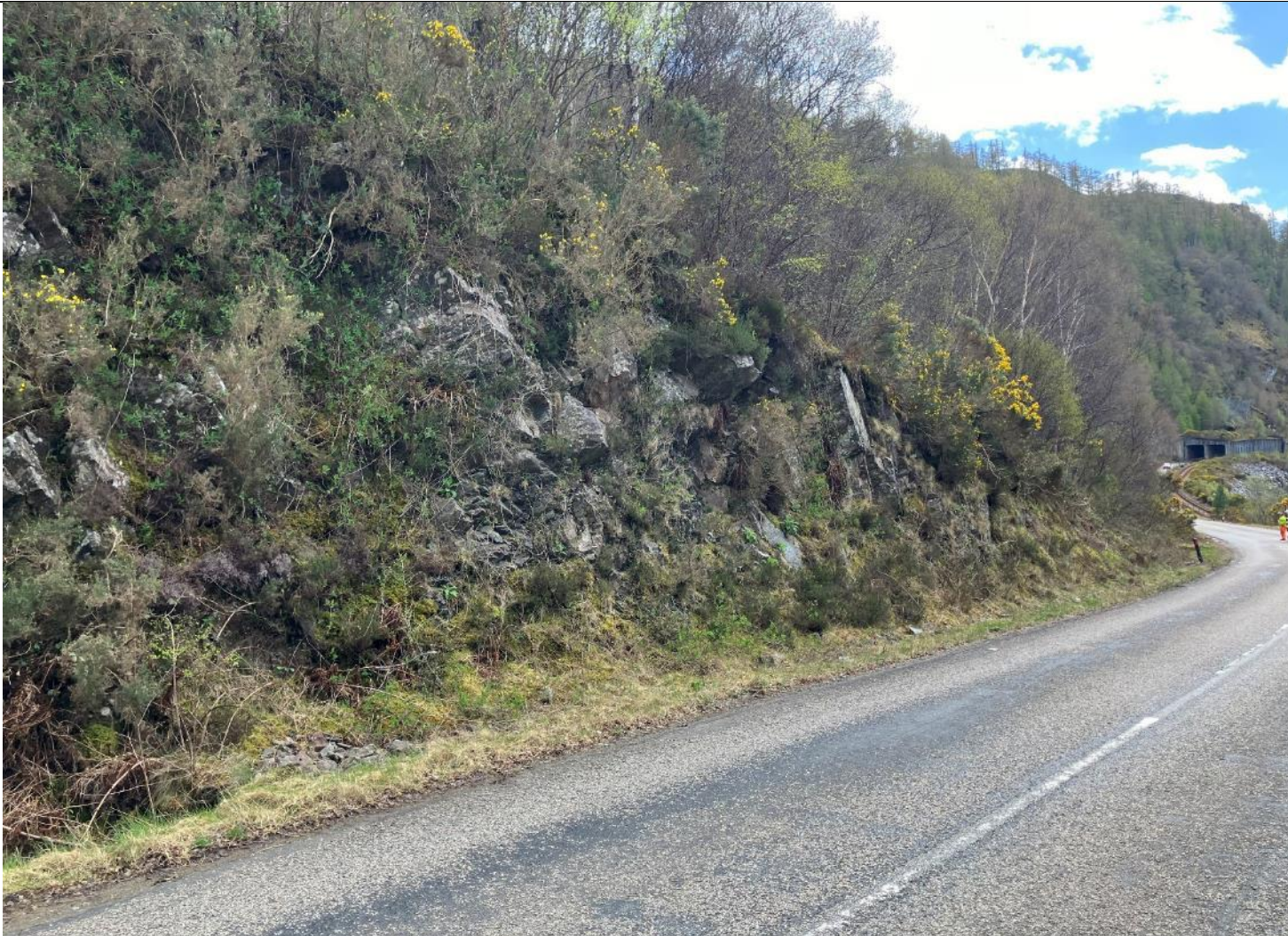
Between Ch. 3655 to 3672 – Potential for small blocks to fall due to ravelling and root jacking.
