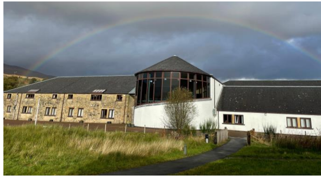
Ardnamurchan High School - located next door to Strontian Primary School
