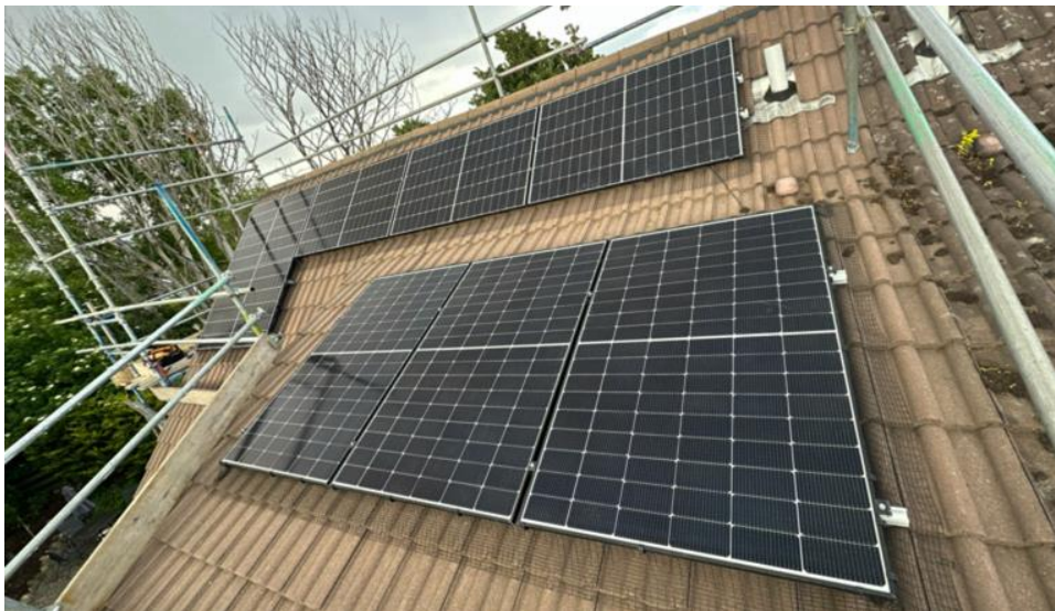
Figure 2 - Solar Photovoltaic panels post install
