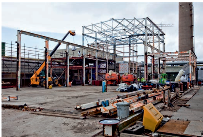
FCA building demolition in progress
