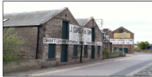
expanding timber processing at Balblair
