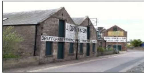
expanding timber processing at Balblair
