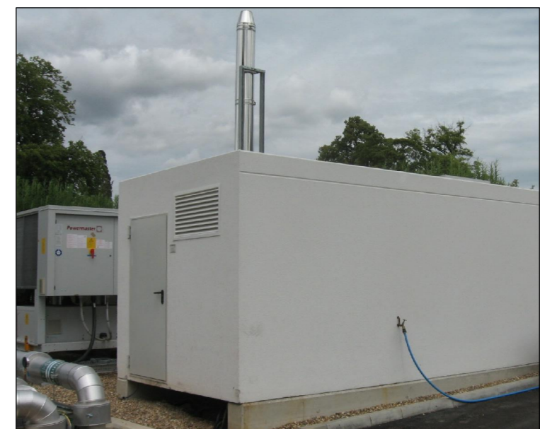
TYPICAL PREFABRICATED BOILER HOUSE EXTERNAL
