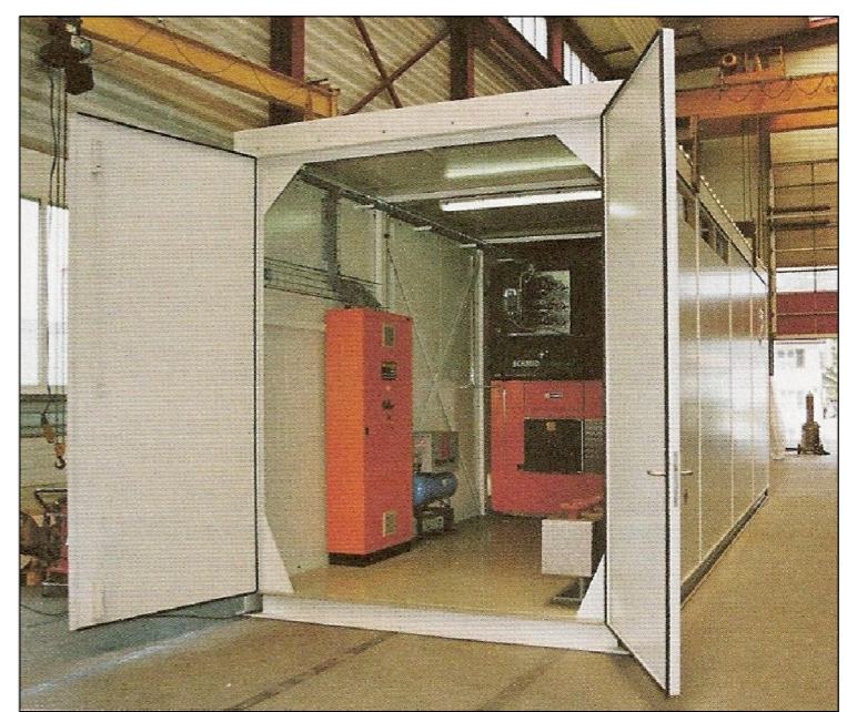
TYPICAL PREFABRICATED BOILER HOUSE INTERNAL
