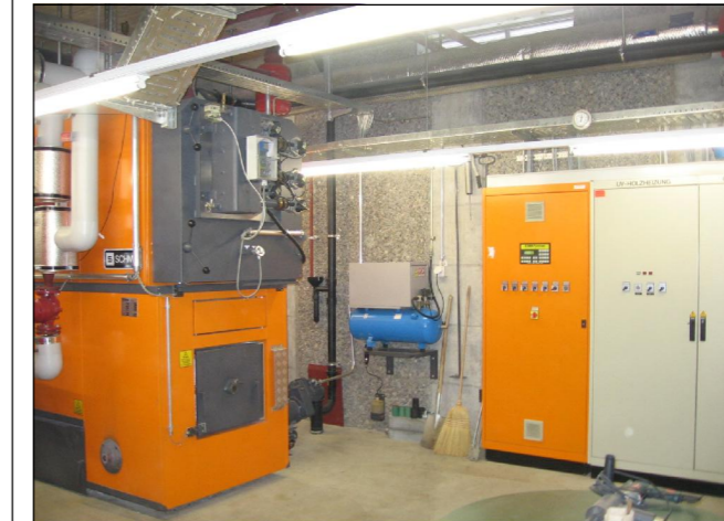
TYPICAL BIOMASS BOILER INSTALLATION
