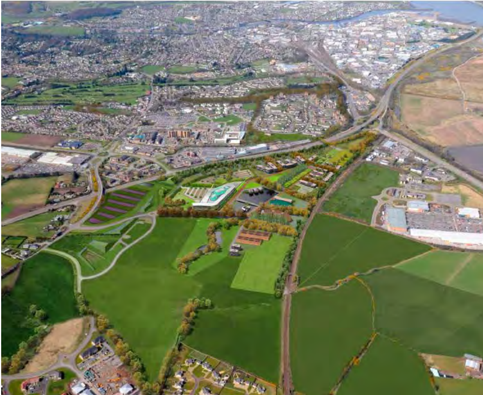
Aerial view of Inverness Campus from East
