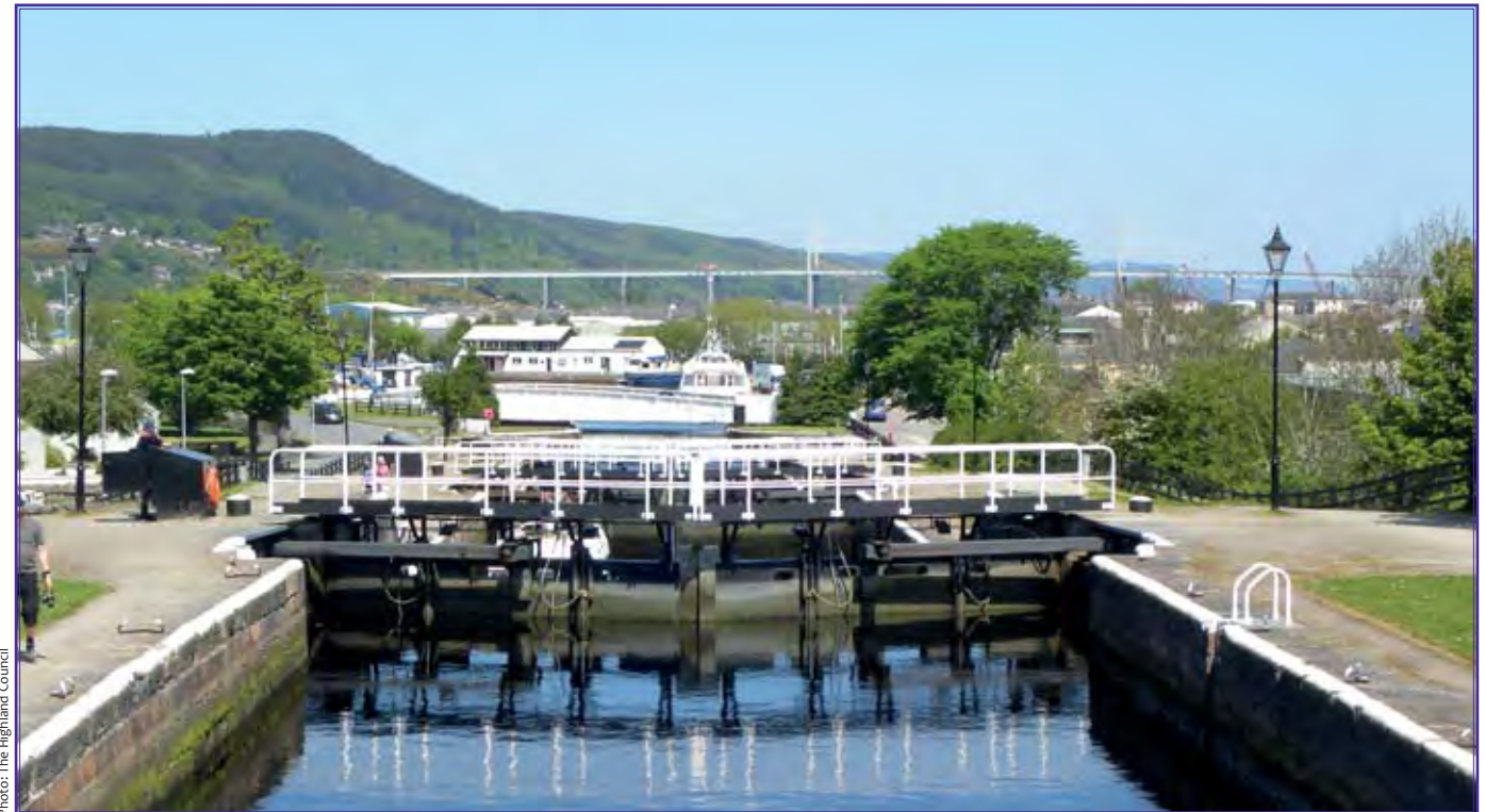
Photo: The Highland Council
