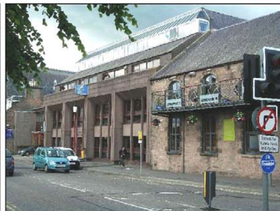
Concrete Frame & Panelling - Moray House - Bank St.
