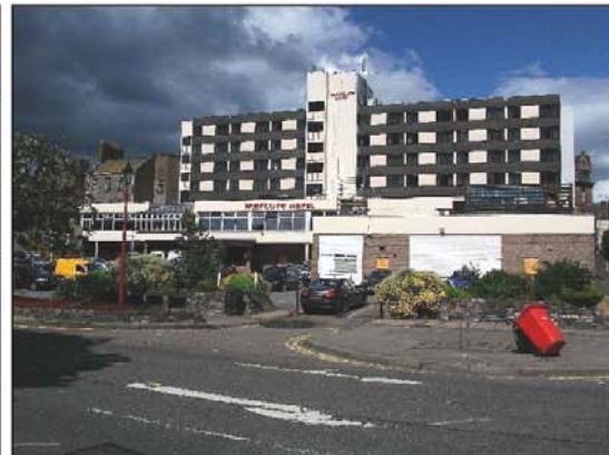
Concrete Frame & Cladding - Mercure Hotel - Bank St. & Church St.
