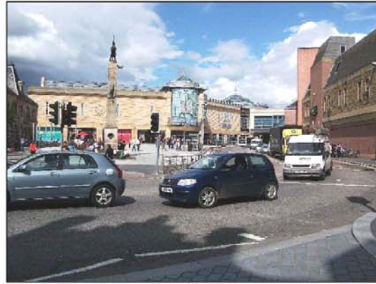
Facing Block / Stone Cladding - Eastgate Shopping Centre - Phase 1 & Phase 2
