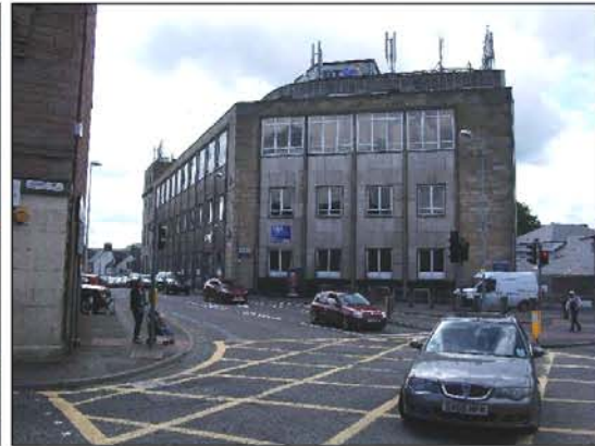
Stone & Panel - BT Exchange - Friars St
