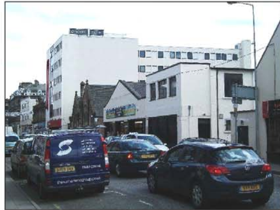
Painted Concrete Panel - Encore Hotel - Academy St
