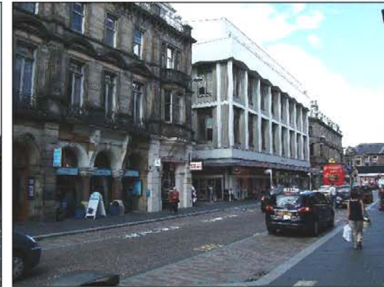
Concrete Frame, Metal Cladding - Post Office - Queensgate
