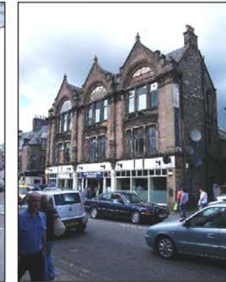
Stone & Slate - Al Welders - Academy St
