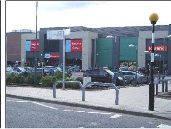
Composite Panel, Steel Roofing - Retail Units - Rose St.
