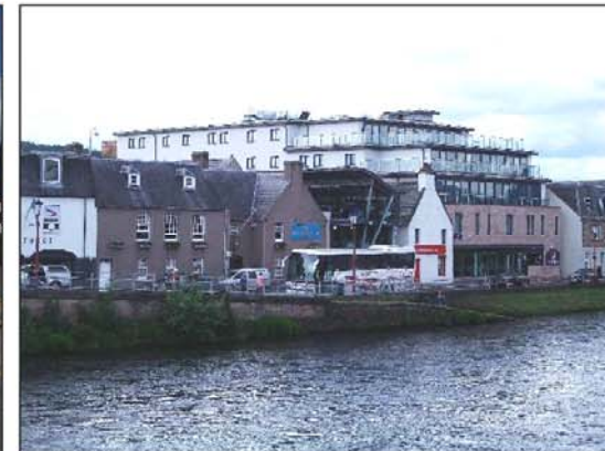
Steel Frame, Render, Stone Facing - Premier Inn - Huntly St.
