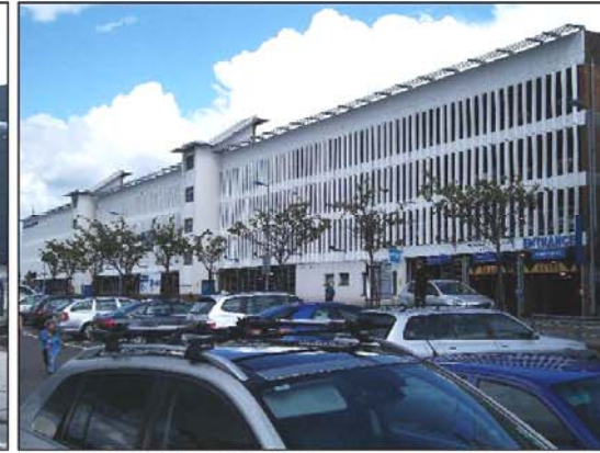
Concrete Frame & Panel - Car Park - Rose St.
