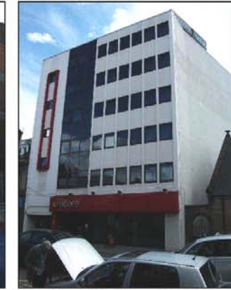
Painted Concrete Panel - Encore Hotel - Academy St
