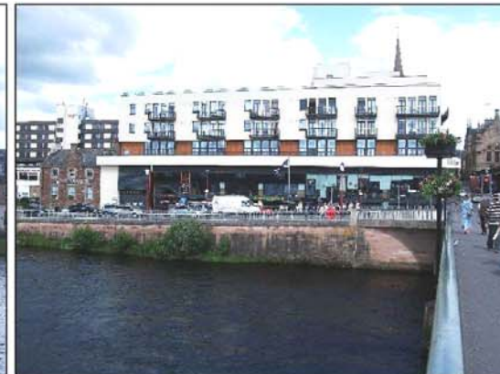
Concrete Frame, Render - Bridge House - Bank St.
