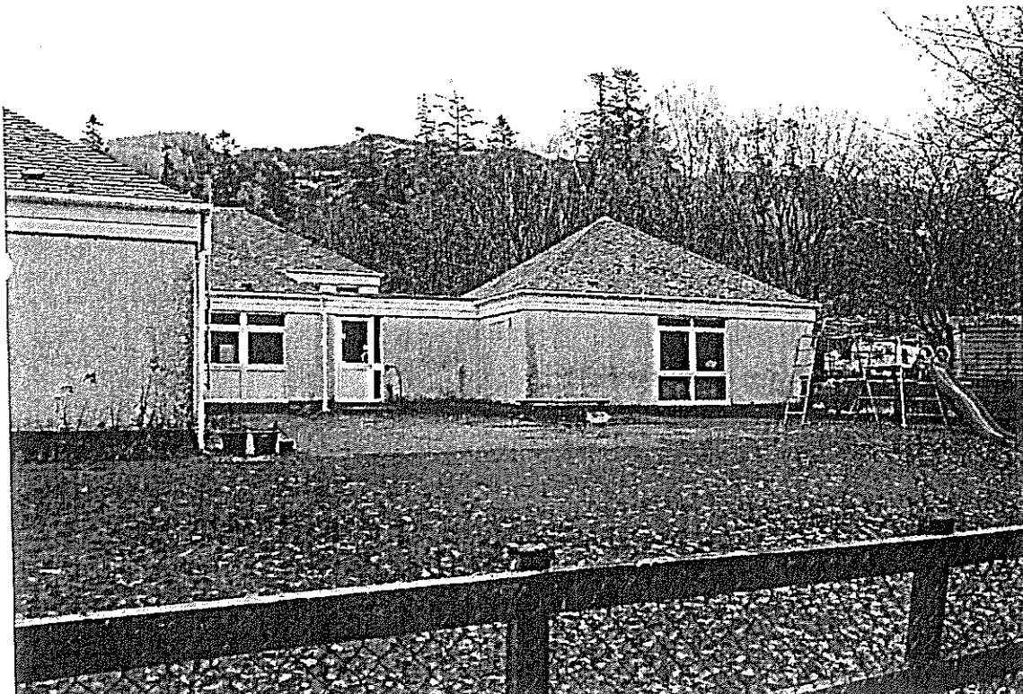
Photo 2. P1 to P3 playground hard paved area.
