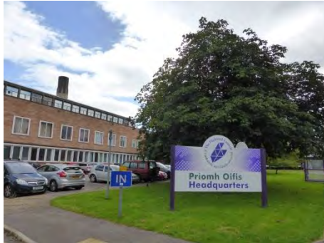
The Highland Council Headquarters
