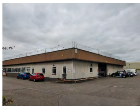
Building Maintenance Depot, Harbour Road
