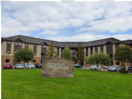
Planning office, Kintail House, Beechwood Park
