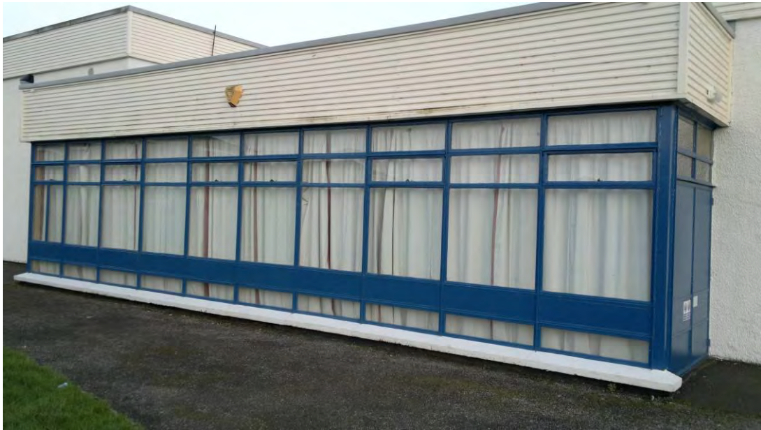
Figure 2 North west façade.
