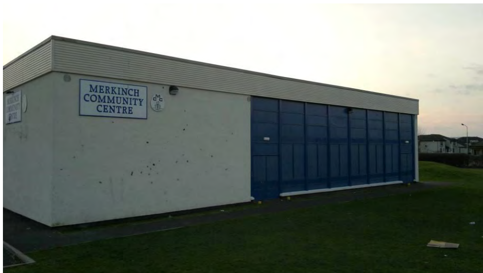
Figure 1 – North east façade showing main hall windows.
