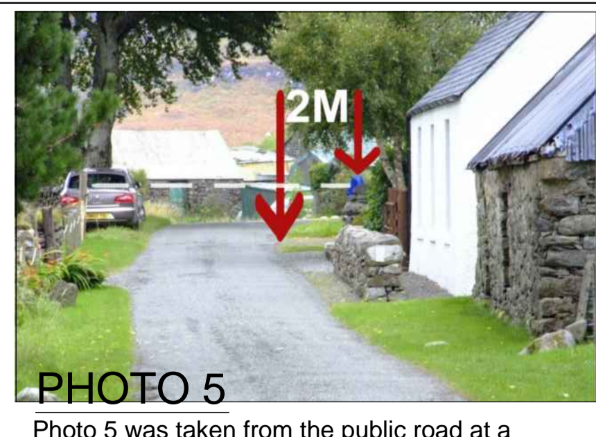
Photo 5 was taken from the public road at a distance of 65M from the proposed entrance. The blue jacket represents the position a drivers head would be at upon exiting the proposed access.
