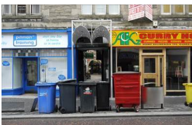
The shop on the left retains its traditional shopfront, while that on the
