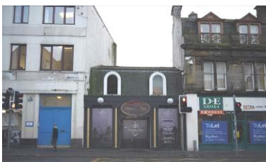
This under-sized infill building at 57 Academy Street means the space still feels like a gap
