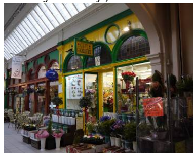
The florist's retains a historic shopfront, with slender colonettes, and attractive clerestory leaded glazing.
