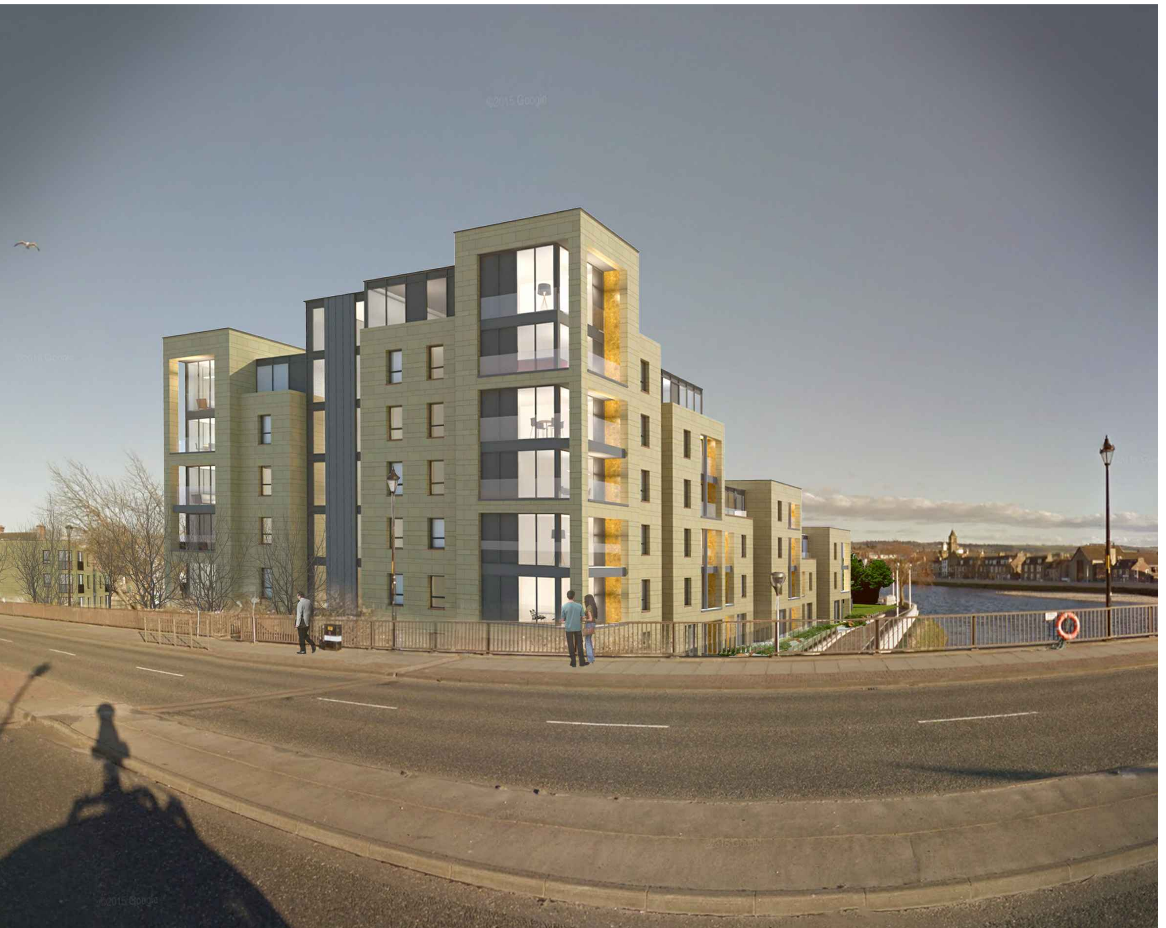
Gateway building at Friars Bridge
