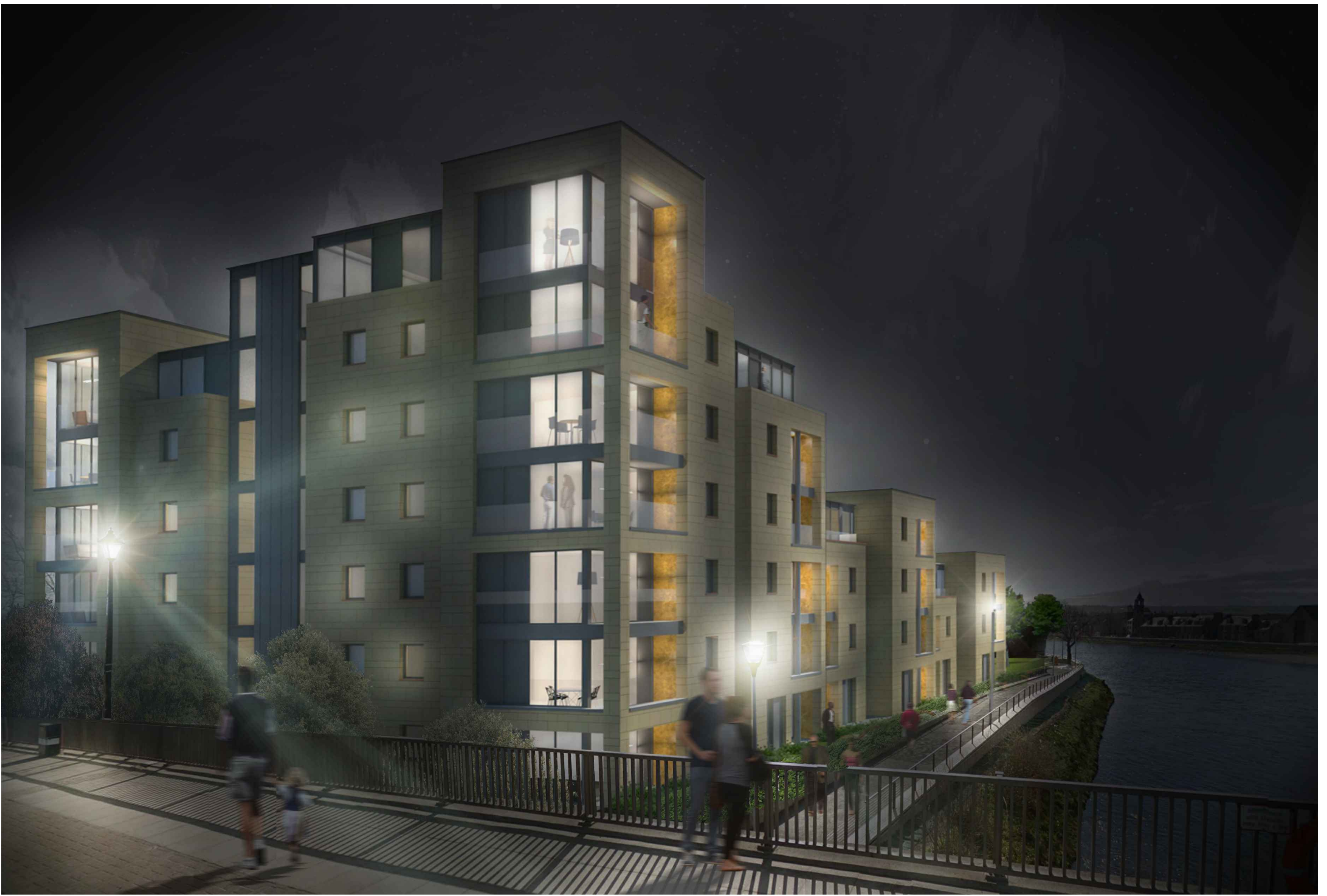
Gateway building at Friars Bridge
