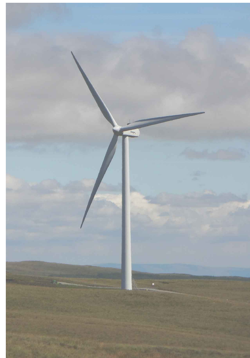
PHOTOGRAPH OF TYPICAL TURBINE
