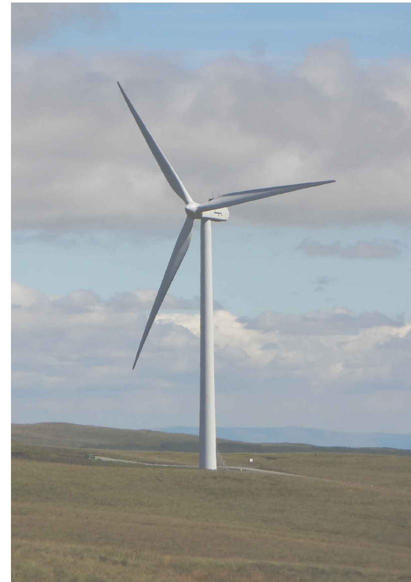
PHOTOGRAPH OF TYPICAL TURBINE
