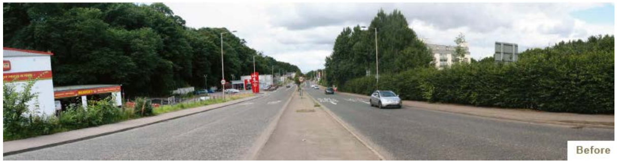
Image 26 – Millburn Road – before
