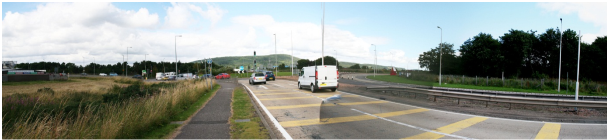
Image 2 – A9 Northbound - before
