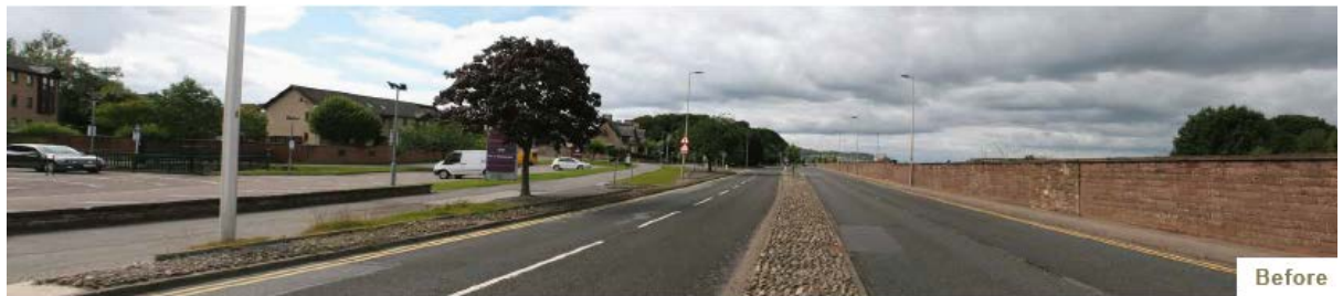
Image 28 – Millburn Road 2 - before
