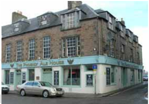
Figure: 7.2 Inverness Townscape Heritage Project Priority Project: 106-110 Academy Street (The Phoenix)
