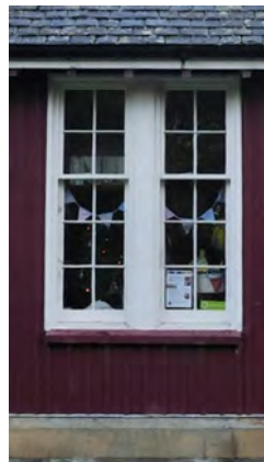
4 over 6-pane sash window.
