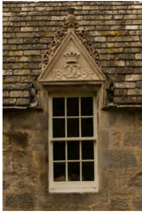
12-pane sash window. Note the slender glazing bars, or astragals.
