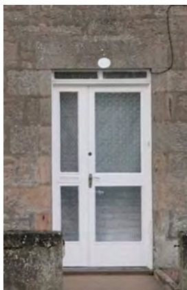
Glazed door with fixed panel. Doors should be made to fit the proportions of the doorway; infill panels are not acceptable.
