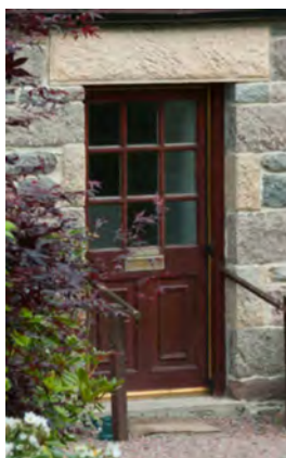
Off-the-shelf composite door with glazing panels lacks the subtlety and quality of finish of a traditional door.
