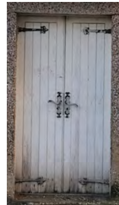
Plank and batten door with attractive cast iron door furniture.
