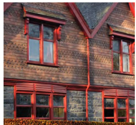
Casement windows with ornate stained glass.
