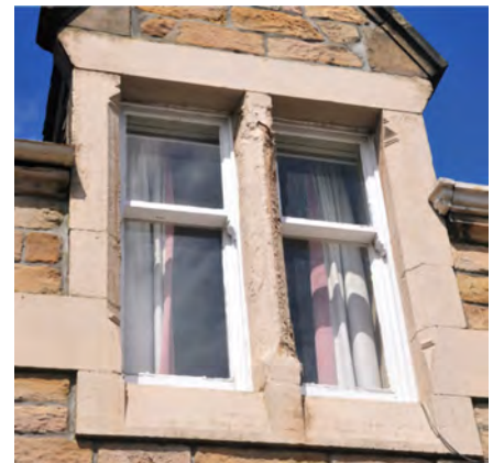
Note how the top sash projects over the lower sash. This example has 'horns'.
