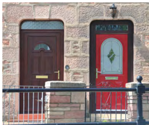
This pair of off-the-shelf uPVC and half glazed doors do not match one another as intended and also detract from the character of the building and wider area.
