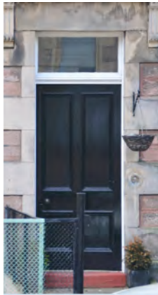
4-panel door with full-pane fanlight, original handle, bell and keyhole.
