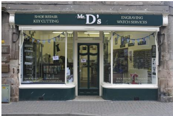
A traditional shopfront, c.1920-30 that, with the exception of the curved glazing to the sides of the lobby, is remarkably intact
