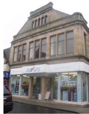
A formerly handsome traditional shopfront that has been replaced by unsympathetic modern design
