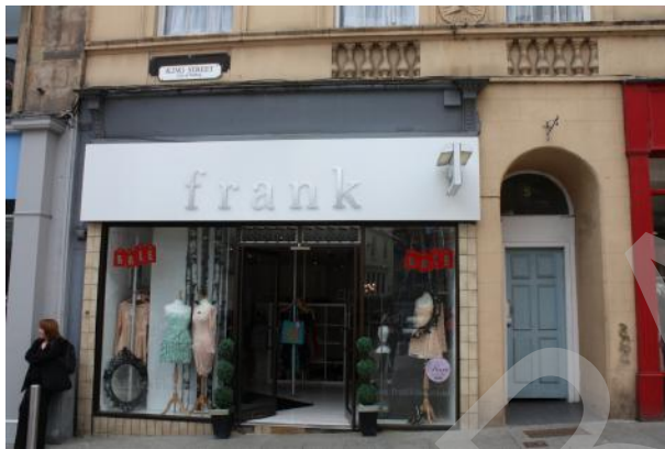
BEFORE: An unsympathetic modern replacement shopfront in a traditional building, King Street, Stirling . Image courtesy of Lindsay Lennie.
