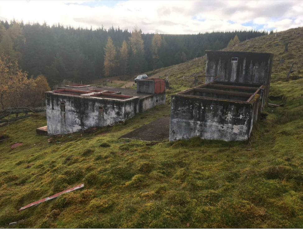
EXISTING REDUNDANT WATER WORKS BUILDINGS
