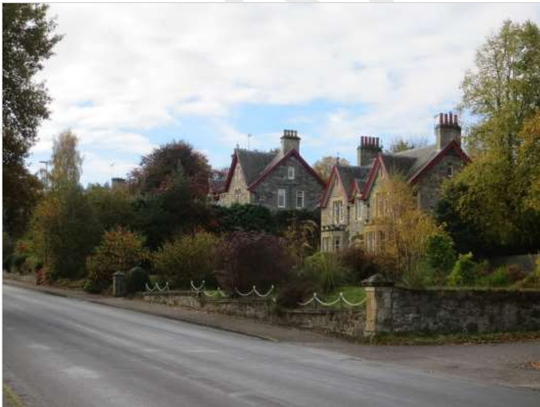
Fig 22: Private gardens in the area surrounding the conservation area contribute to wider green setting
