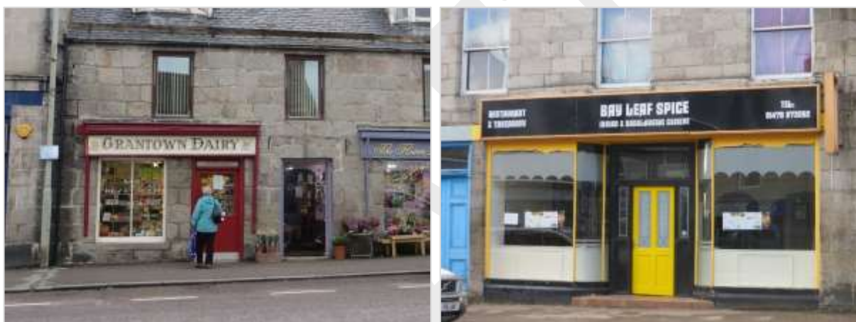
Fig 29: Examples of shop fronts with traditional elements: the Granttown Dairy has a single window and entrance typical of the earliest shop fronts, with sign board and blind box above; the Bay Leaf Spice which has large plate glass window with curved glass and slender colonnades to its entrance.
