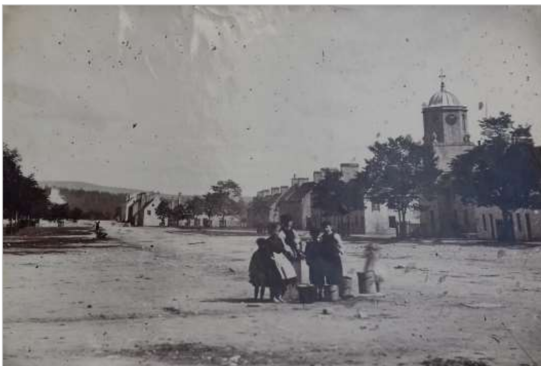
Fig 5B: Early photographic image of the Square (c.1865) showing the Georgian regularity (excepting the landmark Speyside Orphanage) prior to construction of the Court House in 1868 and redevelopment of the Grant Arms hotel. (Urquhart courtesy of Dixon)
