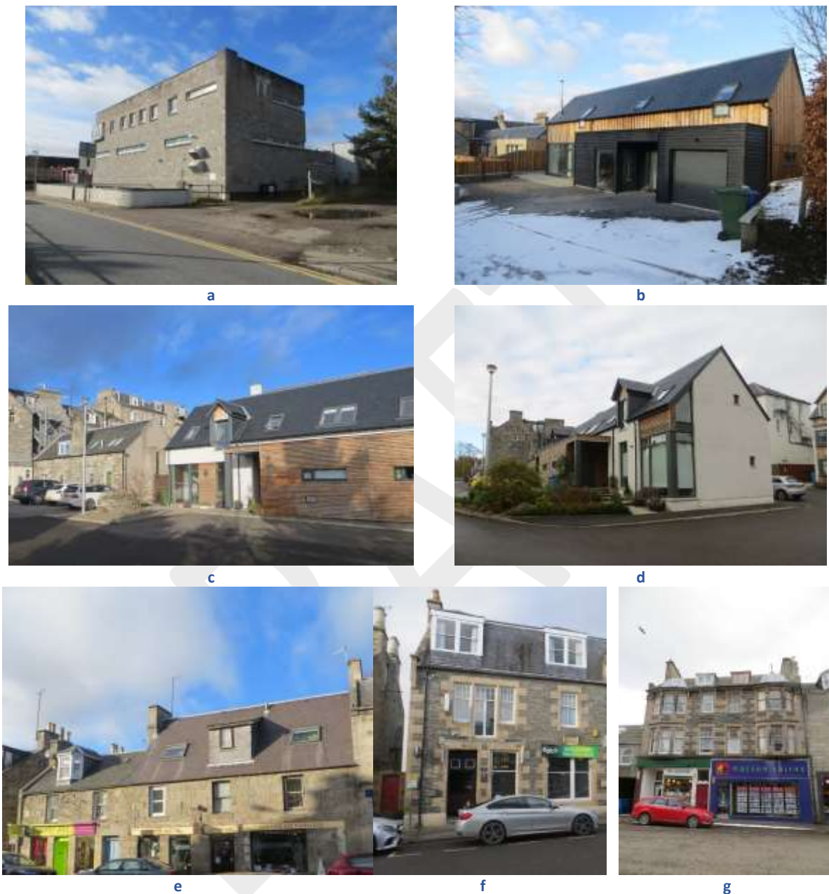
Fig 37: Examples of positive and negative design: the former Telephone Exchange building (a) is not in-keeping with the form and scale of the conservation area; new residential designs which make a positive contribution (b-d); roofscape is important, however large rooflights, box dormers and mansard roofs can detract (e & f); original small rectangular dormers on this Edwardian tenement (g) however the windows on the left dormer have been replaced altering the design intent; the traditional shop front (left) is dwarfed by its neighbour which is not sympathetic to the shop frontage or tenement as a whole.
