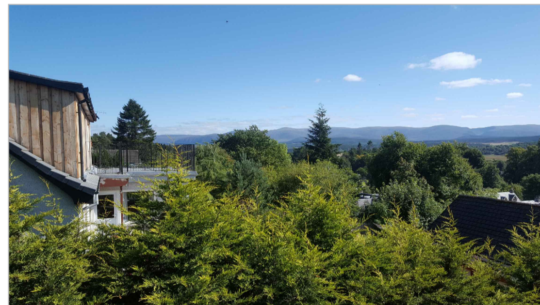
2. Tree screening to the east elevation from First Floor scaffolding
