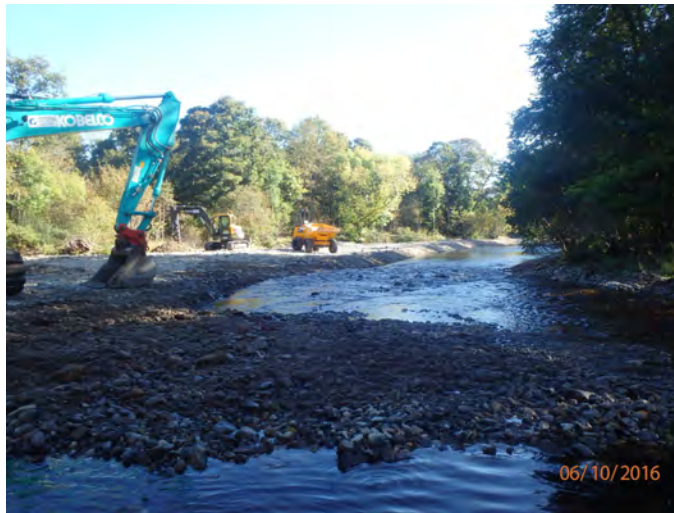
Figure 2-3 - Dredging Works to River Enrick, 2016
