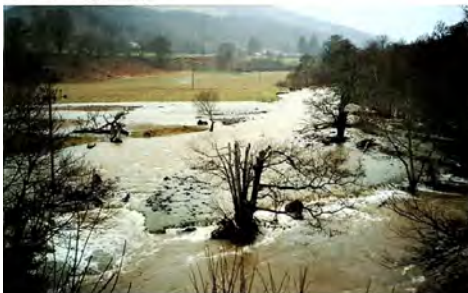
Upstream of AB2 Bridge
