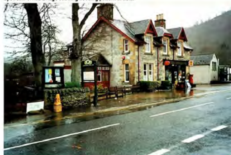
Flooding to Post Office
