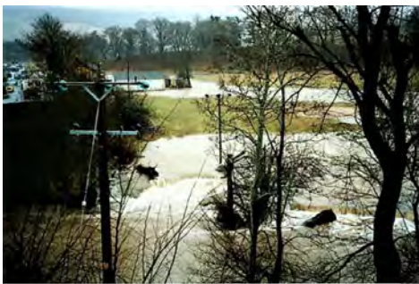
Upstream of AB2 Bridge showing flooding pattern in field.
