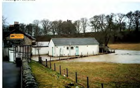
Flooding to rear of Post Office.
