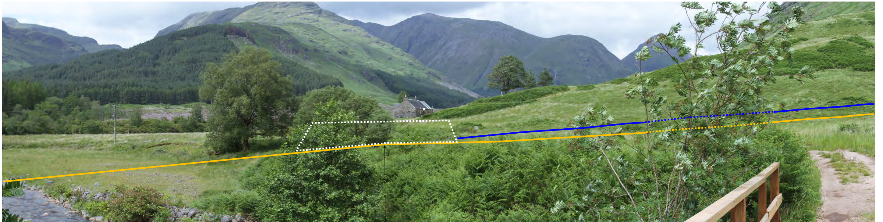
VP9a: Annotated view - Bridge south of Glenceitlein facing north
