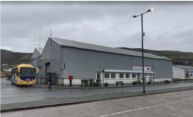
Picture 2.2 Existing terminal building
