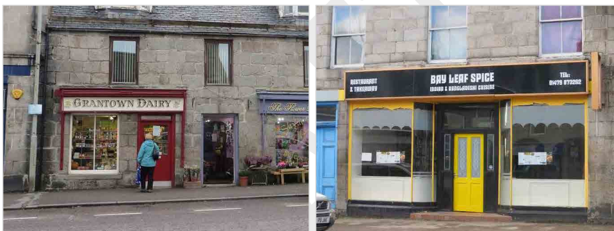
Fig 29: Examples of shop fronts with traditional elements: the Grantown Dairy has a single window and entrance typical of the earliest shop fronts, with sign board and blind box above; the Bay Leaf Spice which has large plate glass window with curved glass and slender colonnades to its entrance.
