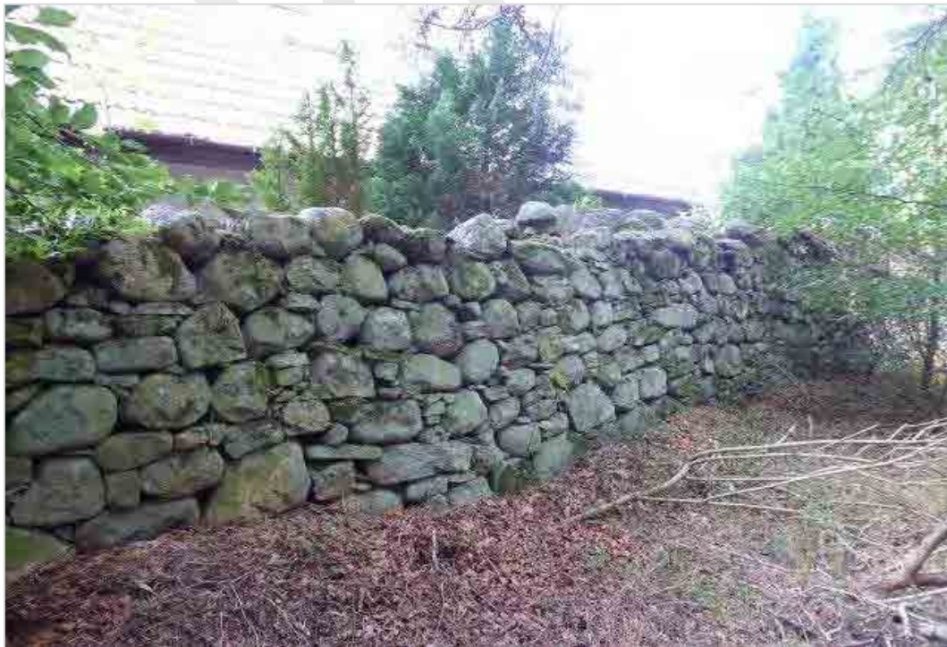
Fig 23 (top): The northern end of Dollar's Dyke at the rear of Pineview with the early outbuilding / stable of the former Free Church manse (now part of Schiehallion Cottage grounds) in the background; (below): large rounded field stones present in the current structure suggest they are original to the 1766 dyke.
