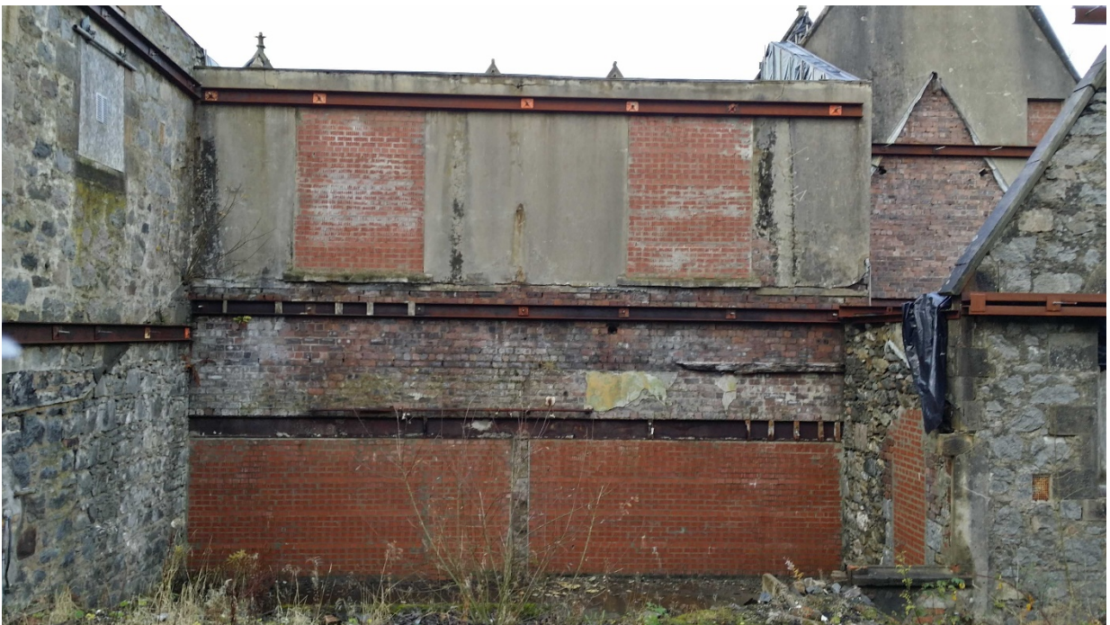
Rear Internal Elevation
