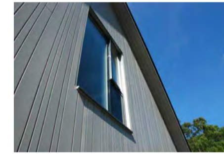
1 - Accoya Timber Cladding Material Key 1 : 25
