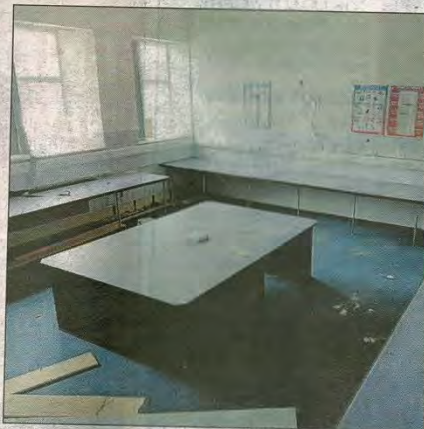
Some upstairs walls will be knocked out.
