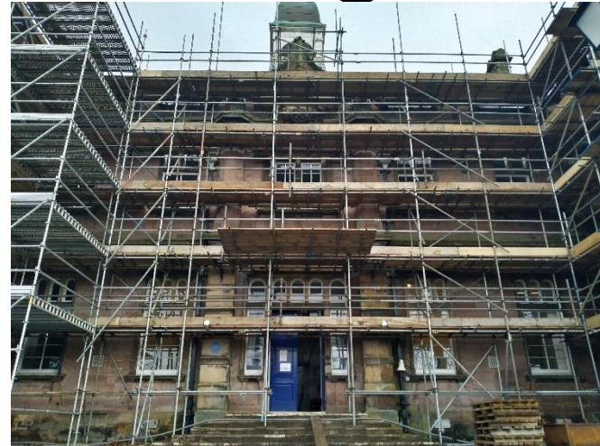
Front / West Elevation Feb 2020
