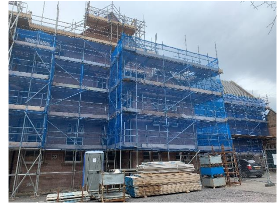
South Elevation March 2020
