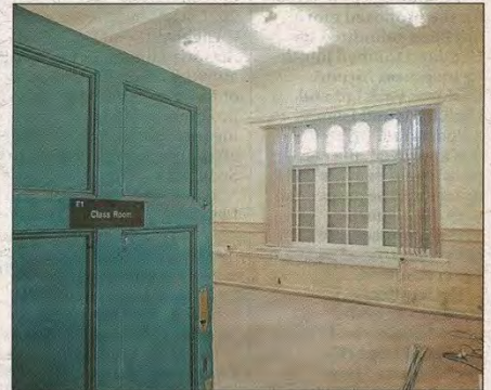
Downstairs classrooms will be converted into offices.
