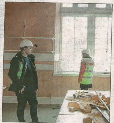
Chris Cowie and Emma Callaghan tour the building.
