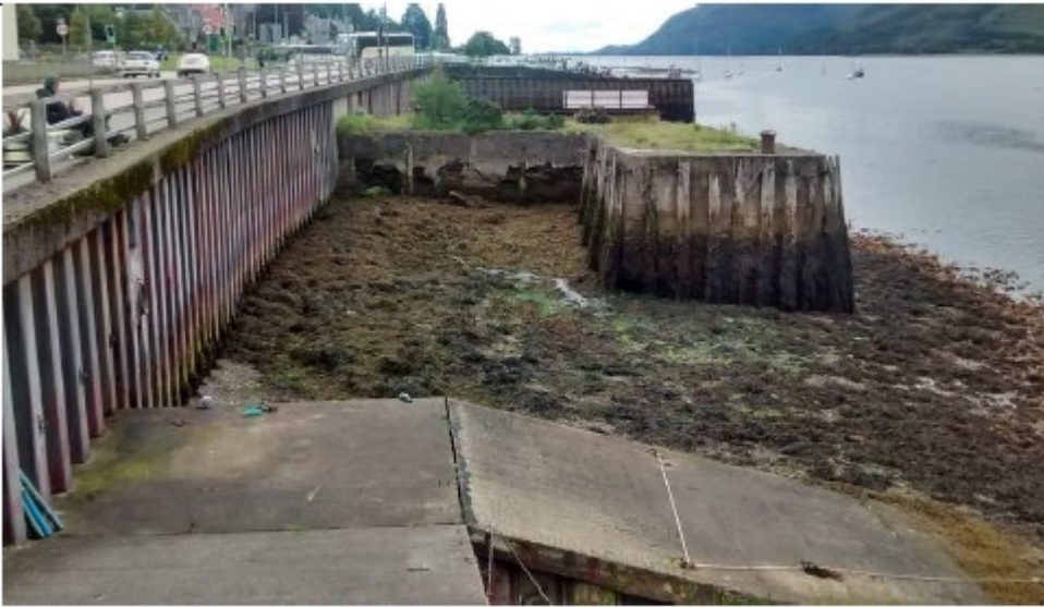
Photograph of area to be filled in and gap where rock armour is to be deposited to keep the dredge material from being washed away
