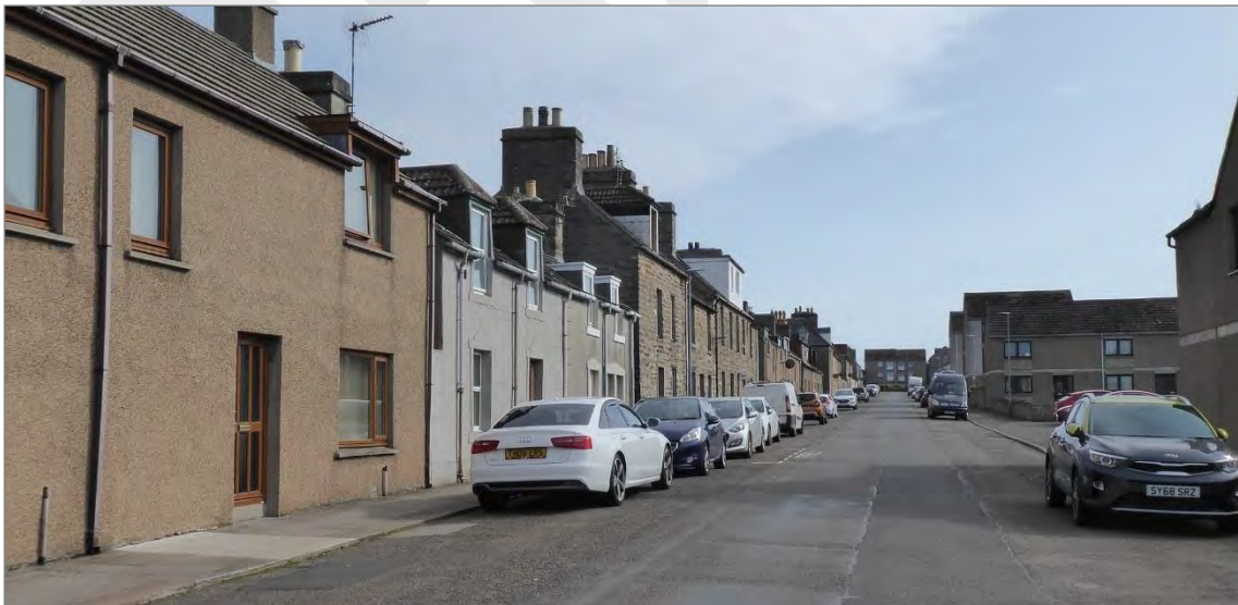
Figure 44: Brown Place: (top) looking east at the turn of the 20 th century with the rope works on the right © The Wick Society - The Johnston Photographic Collection; (below) the same view in 2020.
