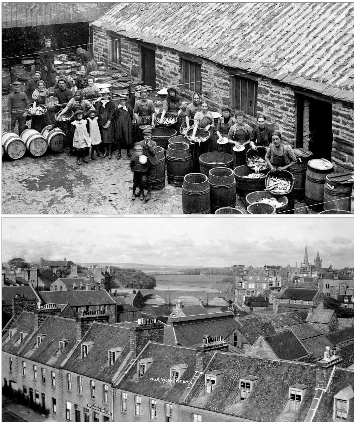
Figure 31: (top) George Cormack’s yard in Lower Pulteneytown in 1900s with pantiles on the roof of the single storey building and what looks to be a Caithness slate easing course at the eaves; a rough cobble stone finish to the yard; (below) Historic view over the roofs in Union Street illustrating the predominance of slate roofing but with other finishes including pantile on some industrial buildings. © The Wick Society - The Johnston Photographic Collection
