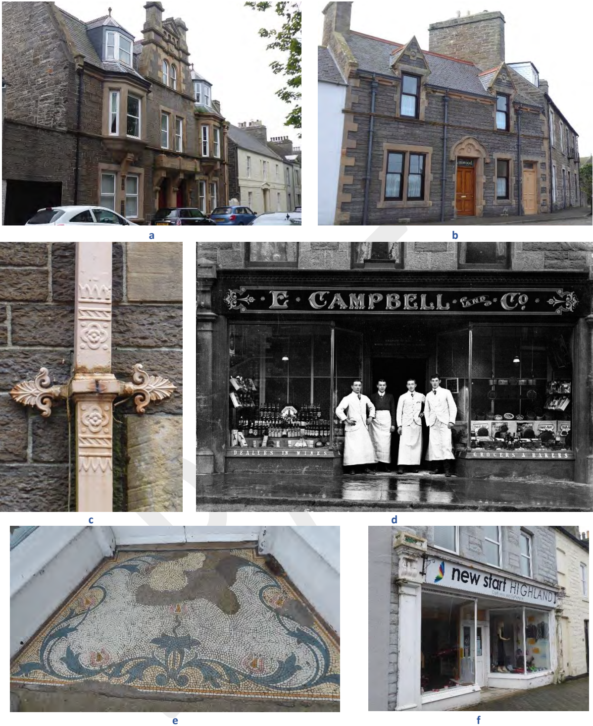
Figure 35: Victorian buildings: a: Nos. 15 and 16 Sinclair Street are elaborate Victorian style houses which dwarf their Georgian neighbours and exhibit much of the change in design and material use by the end of the 19 th century; b: a more modest Edwardian house on Breadalbane Terrace built in 1911 with again more intricate stonework and decorative cast iron rainwater goods; c: decorative square downpipes and acanthus holding brackets at 15 and 16 Sinclair Street; d-f: just out with the conservation area, a late Victorian shopfront survives with a traditional terracotta mosaic entrance platt, originally E. Campbell & Co. Grocers. (Historic image © The Wick Society - The Johnston Photographic Collection).
