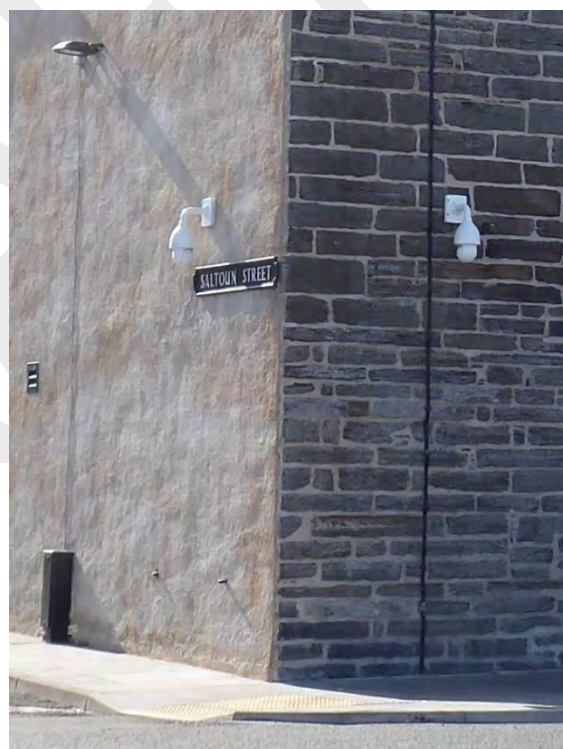
Reinstated lime harling on prominent gable with traditional street sign alongside a standard flood light and two modern white lamps showing a lack of appropriate and coordinated design. Note dropped kerb constructed using textured concrete paving which is not in keeping with the Caithness flagstone.
