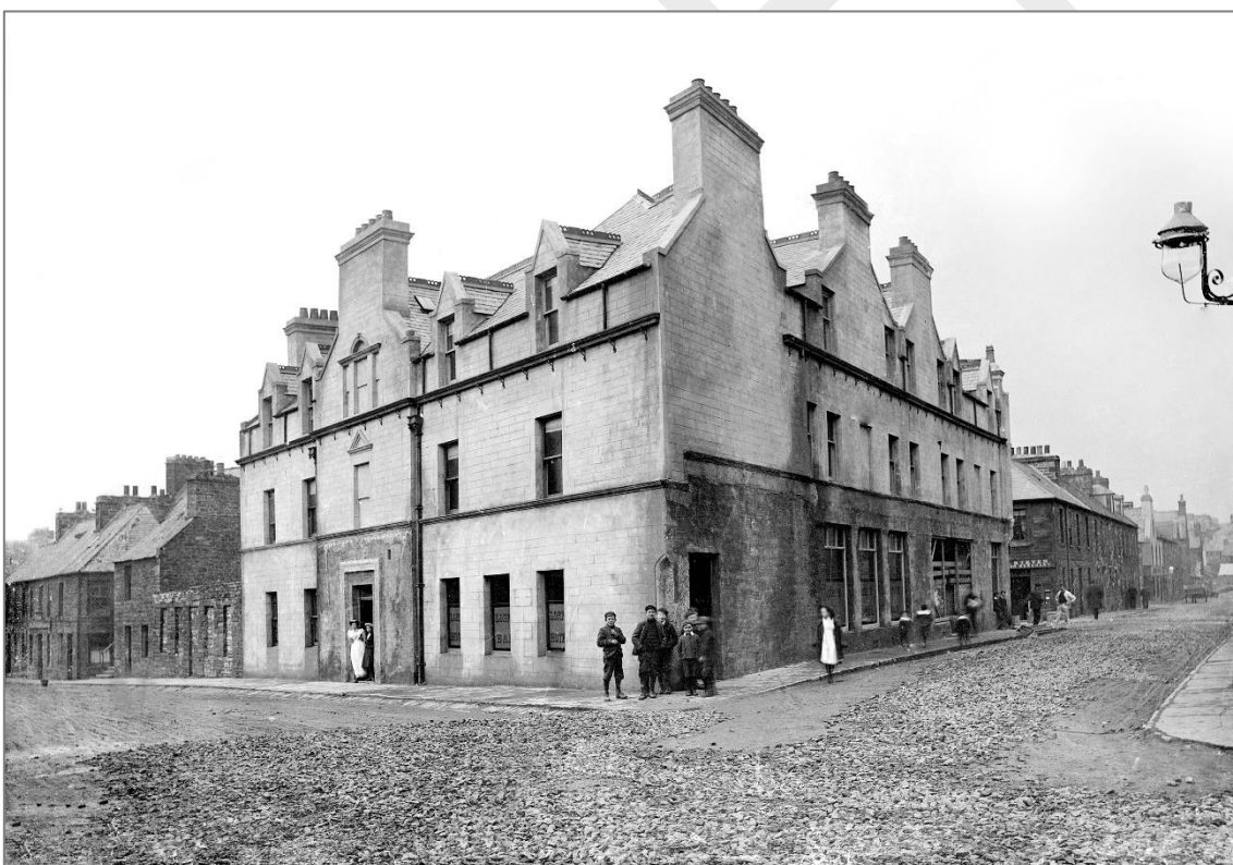
Figure 12: the Lorne Hotel occupied the corner of Bank Row and Williamson Street, pictured here in 1900. In comparison to the redevelopment above, the form and scale of the hotel provided a strong corner and reaffirmation of the urban structure of the industrial area. Note the road surface made up in sea gravel and Caithness stone pavements. © The Wick Society - The Johnston Photographic Collection
