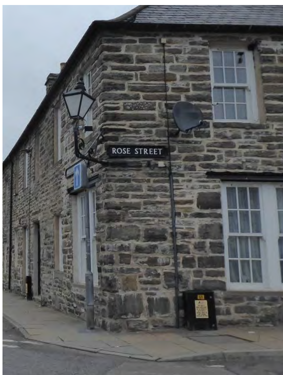
Mixed and cluttered street furniture: enhancement gained by using a traditional lantern and street sign is offset by cabling, satellite dish position and standard one-way road sign. Note the dropped kerb using Caithness flagstone.
