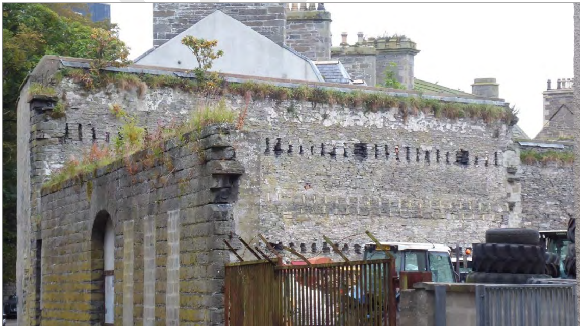
Figure 9: (top) part of the surviving elevation of the former Wick Steam Mills on Union Street with arched opening; (below) masonry side elevation also remaining.
