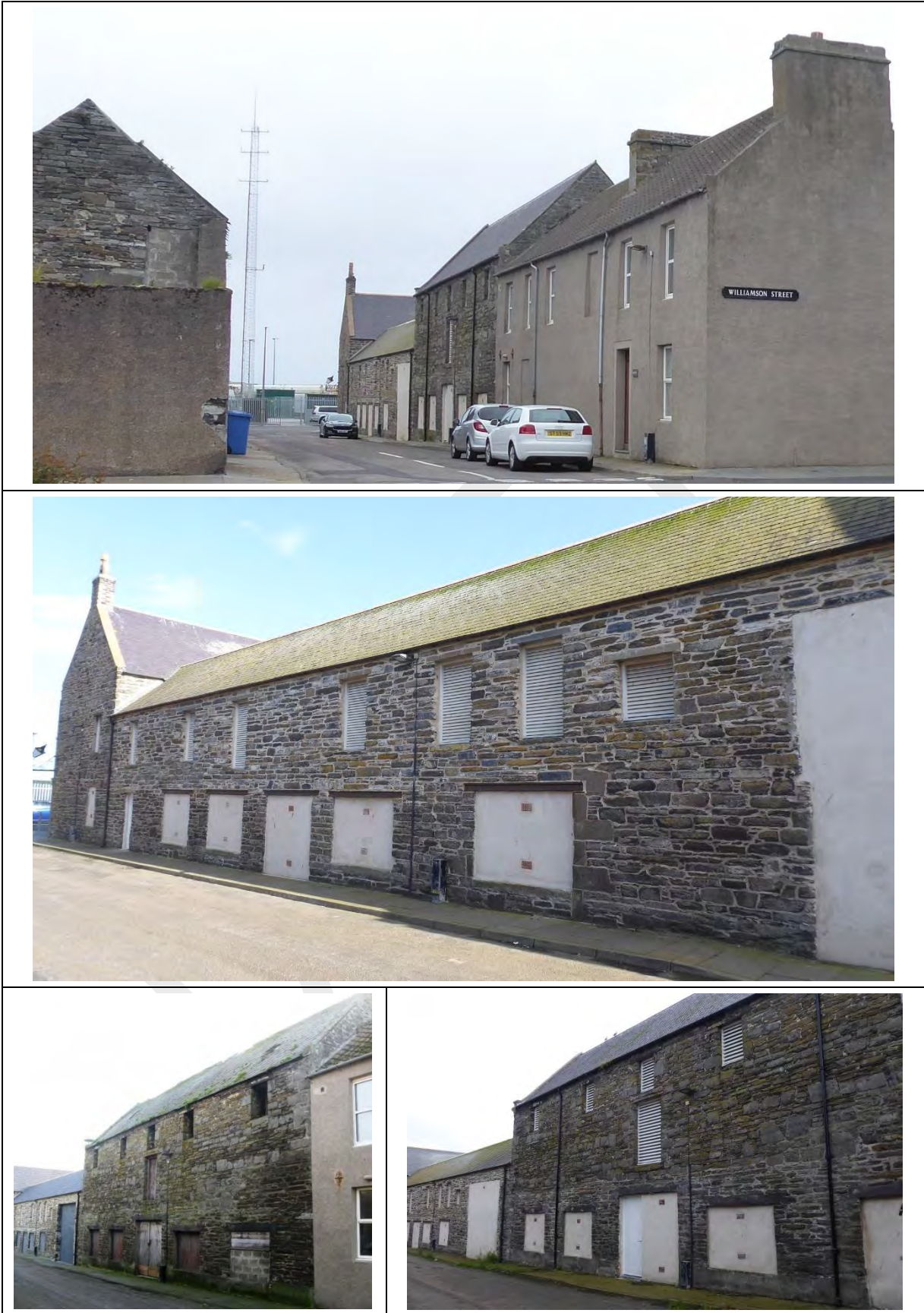
Figure 9: (top) south side of Burn Street looking east to Harbour Quay, 2019; the eastern lots of former curing yard warehouses were repaired in 2012, but still awaiting a new use; (bottom left: BARR 2013 © HES) an early herring house partly repaired sometime after 2013, also vacant.
