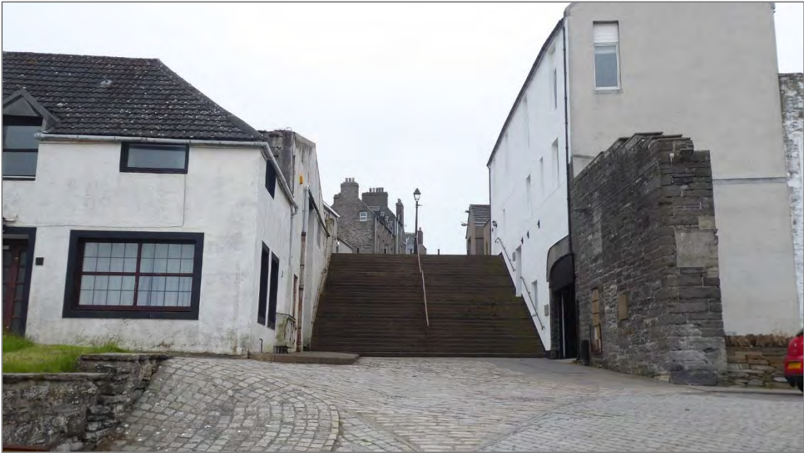
Figure 9: the foot of the Black Stairs, note previous inappropriate alterations to the traditional building on the left (horizontal windows, painted masonry, concrete tile roof); enhancement works as part of previous investment has reintroduced traditional street finishes.
