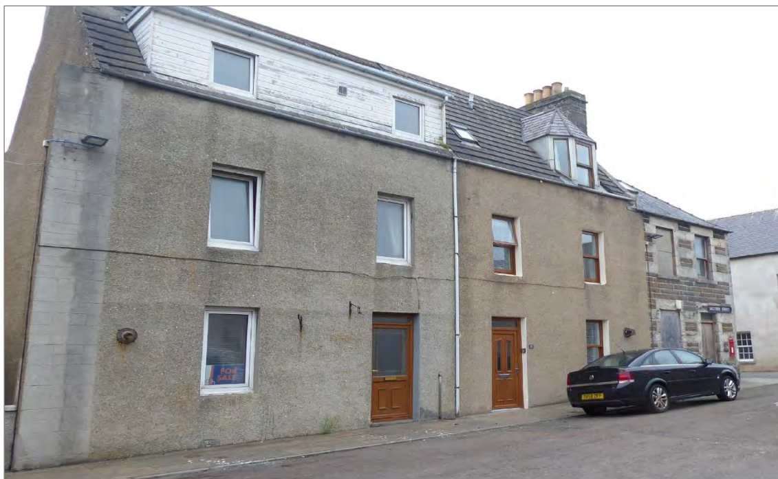
Figure 10: Inappropriate alterations: an example of past unsuitable change to a traditional building of heritage value which results in a negative impact. The original Caithness stone has been covered by a modern cement finish, the original windows and doors have been replaced; the window design and opening method has been altered; a large box dormer has been constructed which changes the form of the roof and obscures the original pitched slope; the original slate finish has been replaced in concrete tile. Buildings such as this can be enhanced and restored when opportunities arise through planning management.
