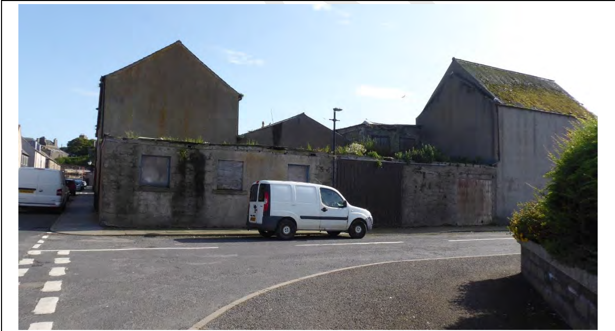
Figure 12: single storey structure on the SW corner of Burn Street and Williamson Street
