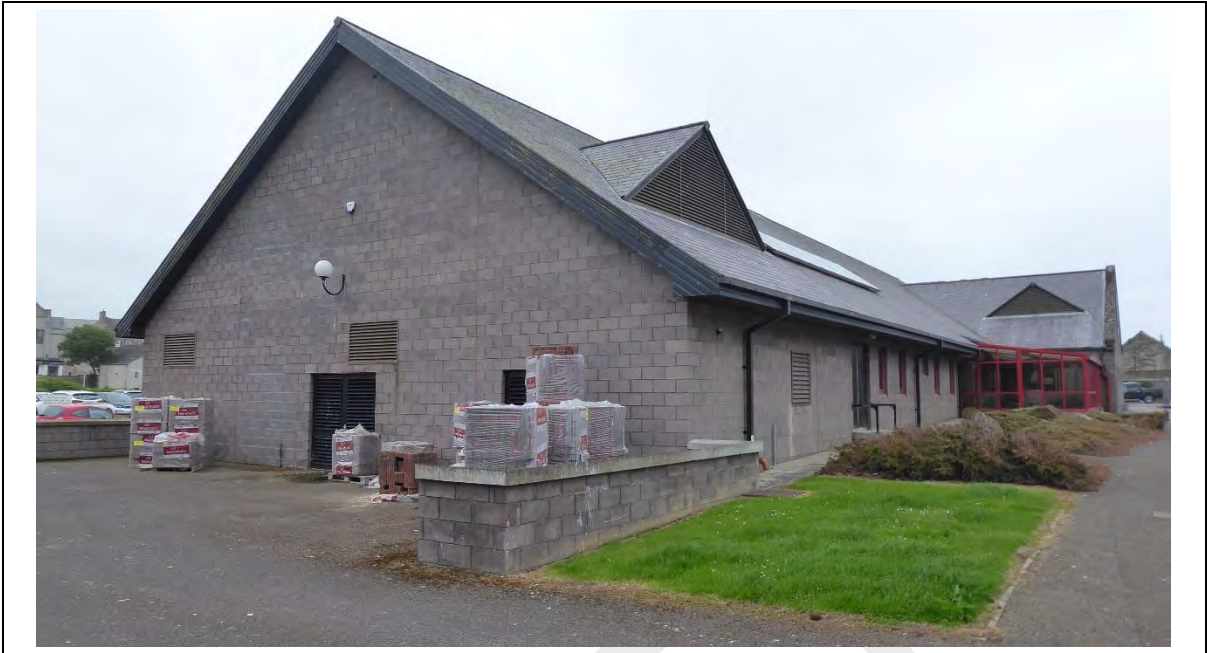
Figure 13: former swimming pool now redundant
