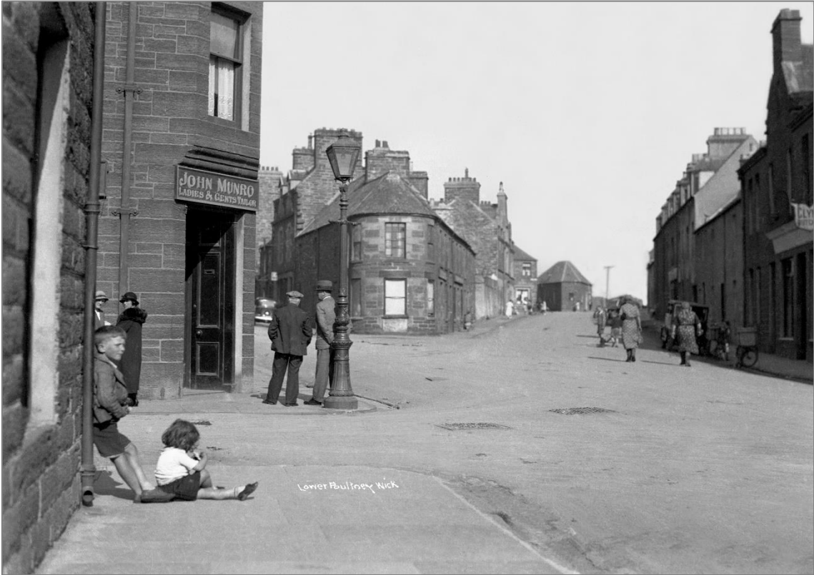
Figure 5: looking east to Bank Row in the 1930s, with the triangular block on Saltoun Street on the left and the former police station building at the end of the boat yard site in the distance. © The Wick Society - The Johnston Photographic Collection ref JN20335B004
