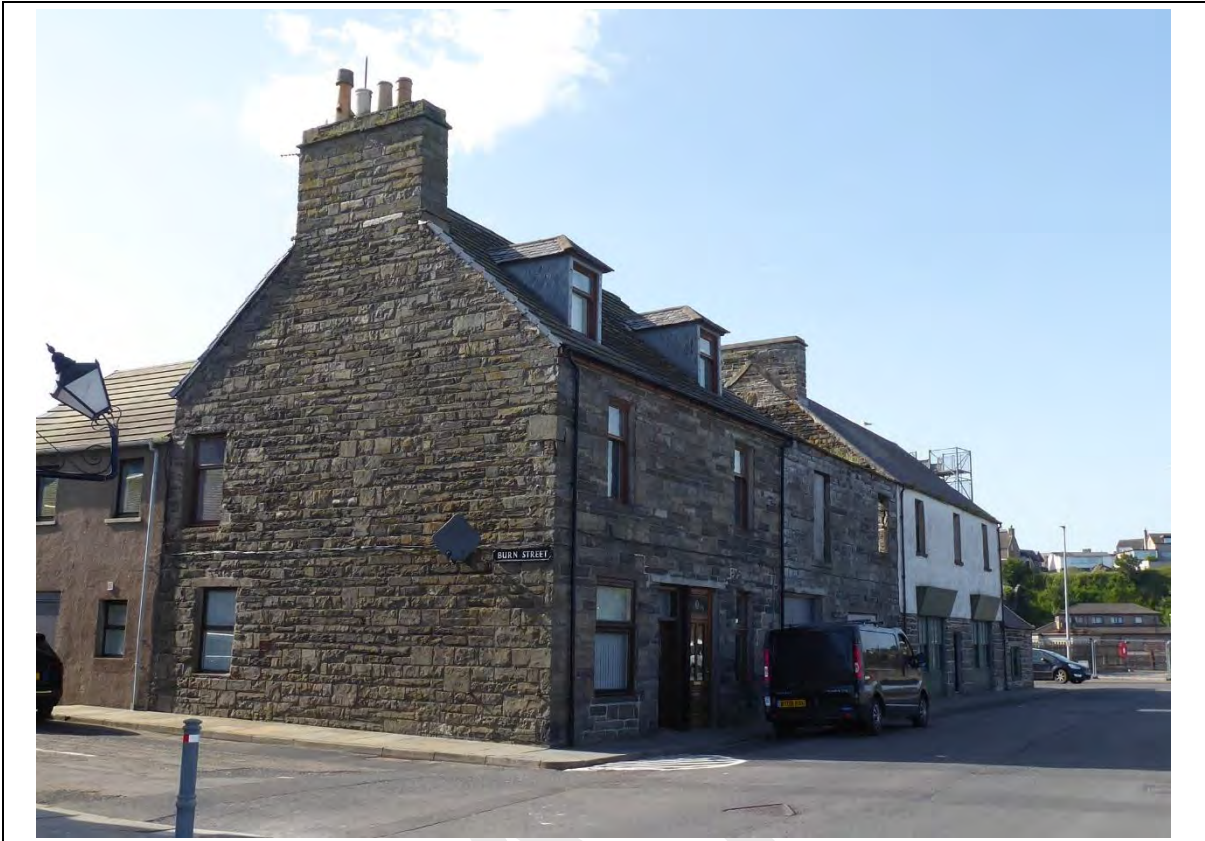
Figure 11: Gap site with surviving façade on Harbour Quay
