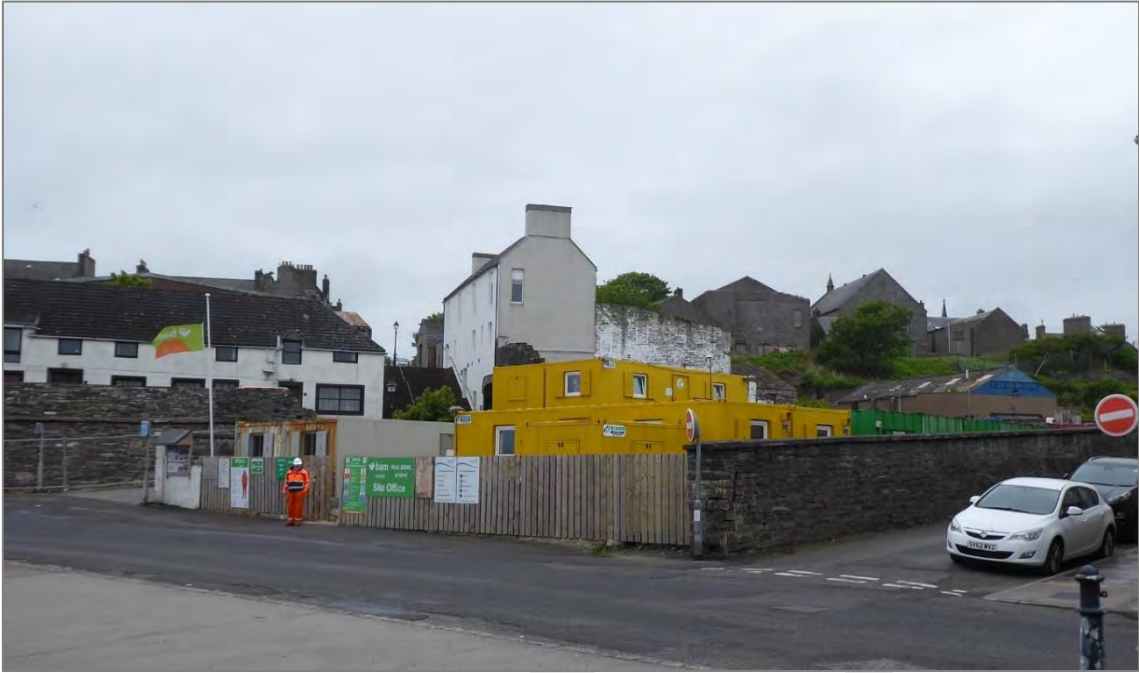
Figure 11: general view of the site in 2019 before the Beatrice construction site cabins were removed.
