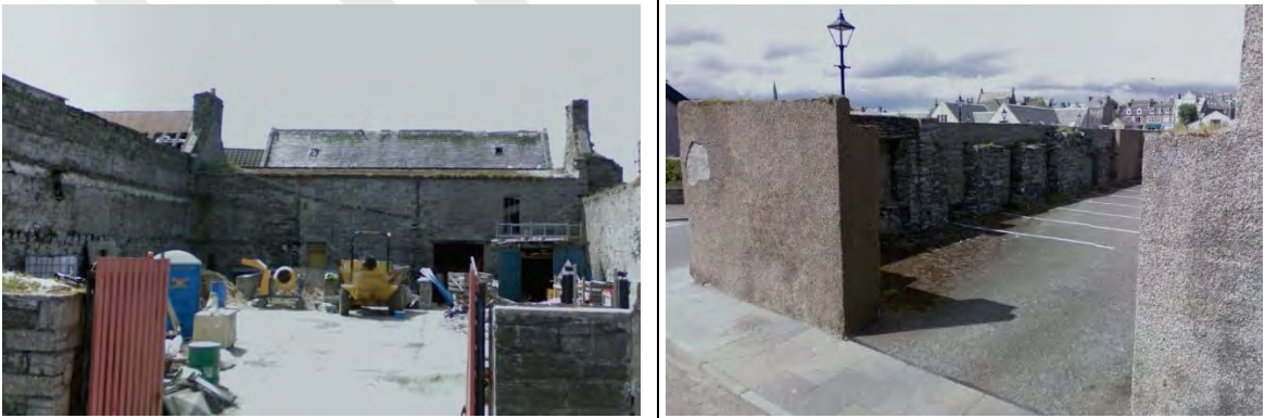
(Above left): potential gap sites include the yard next to GMR Henderson retaining high stone walls defining the original lot; the rear elevation of the de-roofed building on Burn Street is visible at the rear (image 1974 © HES); (right) remains of original Caithness stone walling on the internal face of the boundary wall on Williamson Street (betw. Burn Street and Martha Terrace).
