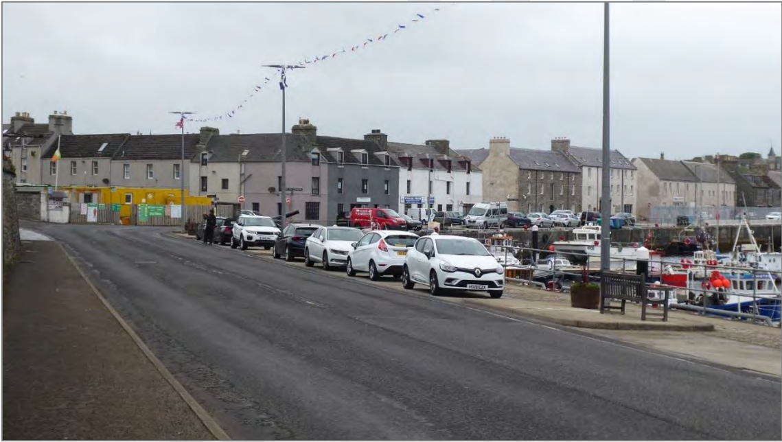
Figure 12: view of the site on approach from the east, the site is highly visible in the important Harbour Quay vista.
