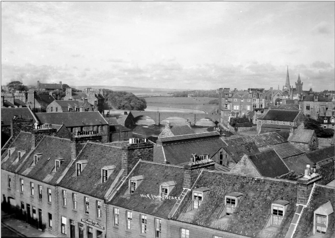
Figure 7: Historic view over the roofs in Union Street illustrating the predominance of slate roofing and also the original building forms with long double pitched roofs extending at right angles to the Union Street frontage. © The Wick Society - The Johnston Photographic Collection. Note kippering kiln with its distinctive ventilator.
