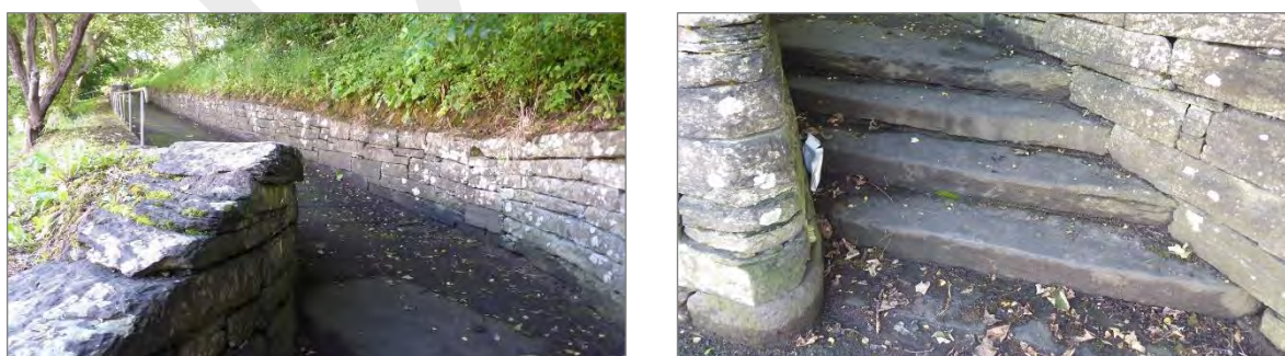
Fig 15: the well-established route across Academy Braes, leading to the upper town, and originally Pulteneytown Academy (now the Assembly Rooms); the original Caithness stone walling and steps remain although the former rough shingle path has been tarmacked with a standard modern metal handrail fitted. A management plan for this green space should include architectural features such as the walling and steps and plans for their retention, maintenance and future repair using appropriate materials and methods. Whilst the green space is semi-natural (rather than a formal landscape) it is very overgrown.
