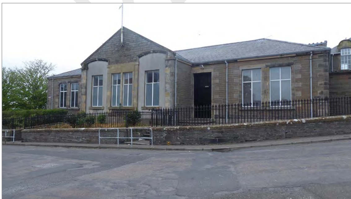
Figure 9: Inappropriate alterations: the importance of retaining architectural detail can be illustrated by comparison of the historic image of Assembly Rooms on Sinclair Terrace and its form in 2019. Constructed as the Pulteneytown Academy in 1838, stripping the building of its architectural features has removed much of the building's original character. Note historic image shows original 'sea gravel' on road and Caithness stone pavement and kerb. © The Wick Society - The Johnston Photographic Collection.
