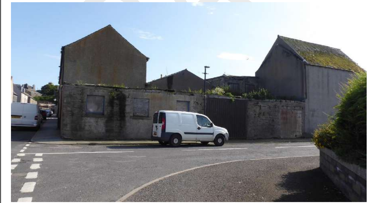
Figure 12: single storey structure on the SW corner of Burn Street and Williamson Street
