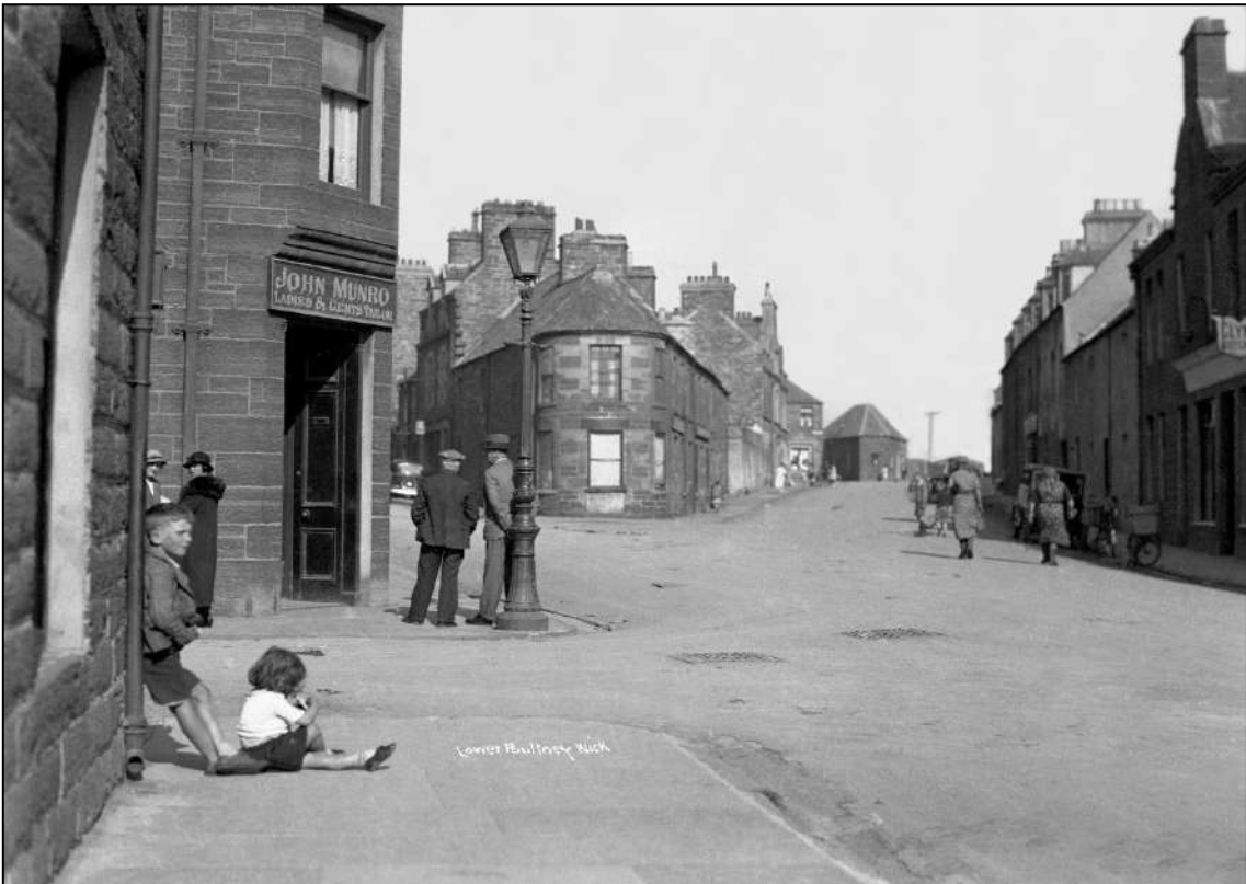
Figure 5: looking east to Bank Row in the 1930s, with the triangular block on Saltoun Street on the left and the former police station building at the end of the boat yard site in the distance. © The Wick Society - The Johnston Photographic Collection ref JN20335B004
