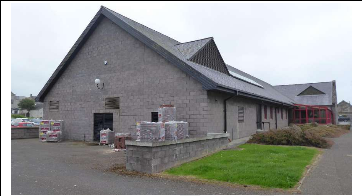
Figure 13: former swimming pool now redundant
