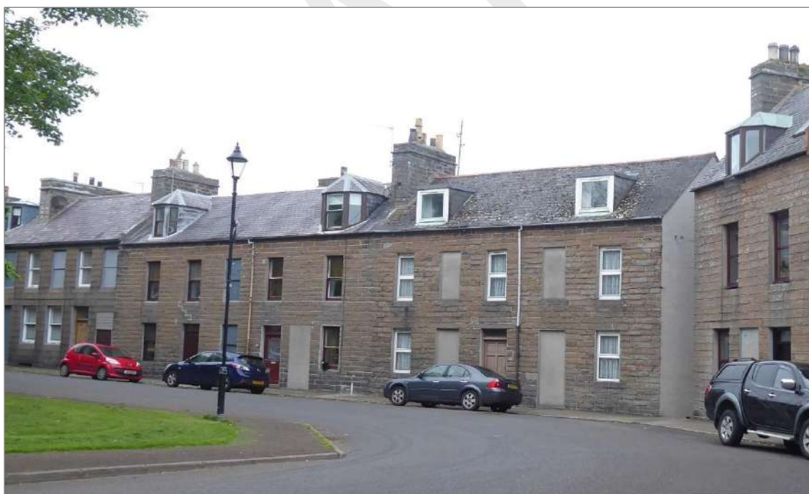
Figure 20: Argyle Square: note the variation on the height of the windows to the eaves, and also the height of the eaves line, which is slightly different between lots.
