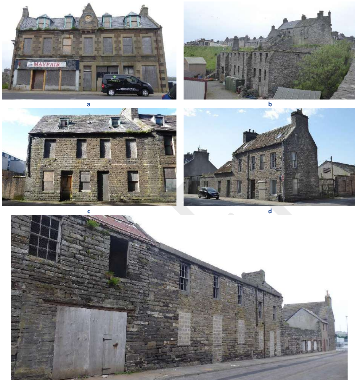
Fig 49 a: former Cooperative store at Nos. 1-4 Macarthur Place (not in CA); b: former Cooperative bakery, South Quay (not in CA); c: Nos. 15 & 16 Union Street; d: No. 2 Union Street; e: partially roofed buildings on Burn Street.
