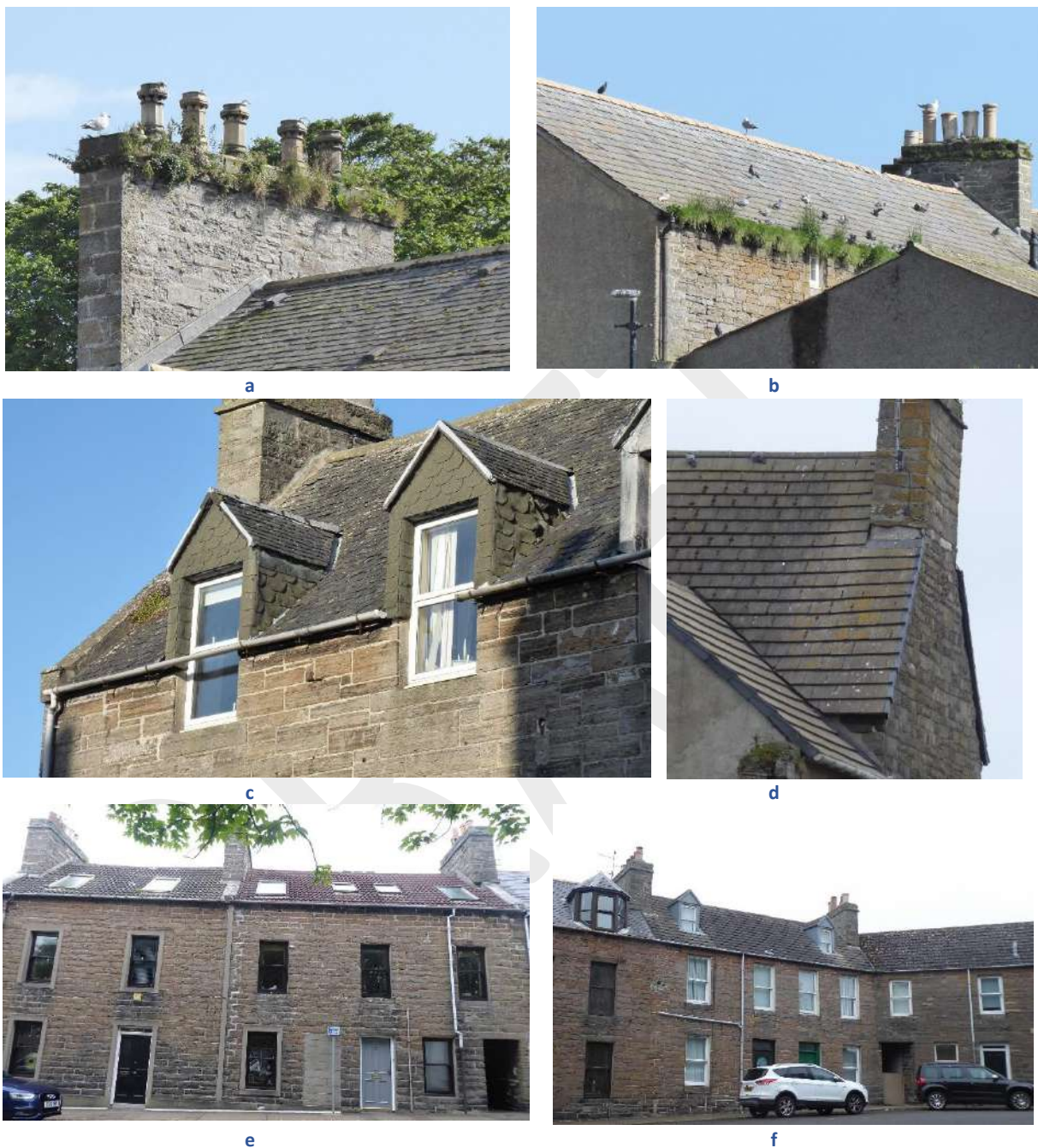
Figure 36: two common examples of vegetation growth leading to different defects and courses of action: a: plants taken root in open mortar joints in the masonry chimney. This is significant and roots unattended will continue to grow into the masonry and expand, over time destabilising the chimney stack; b: grass growing in a presumably blocked gutter with debris forming a soil for the vegetation. Here the blockage will lead to dysfunction of the rainwater system and overflowing of rainwater over the masonry walls and potentially backing up under the roof slate into the interior of the building; c: inappropriate materials, felt tiles, applied to two traditional gabled dormers; d: concrete tile replacement roof with possible removal of stone copes at the gable wall head, replaced by a plastic edge trim; e & f: inappropriate tile roof replacements on the terraced rows in Argyle Square; e: two different tiles, one red in colour both with large replacement rooflights; f: again two different tile finishes with a new slate finish on the left and a later large canted bay dormer.
