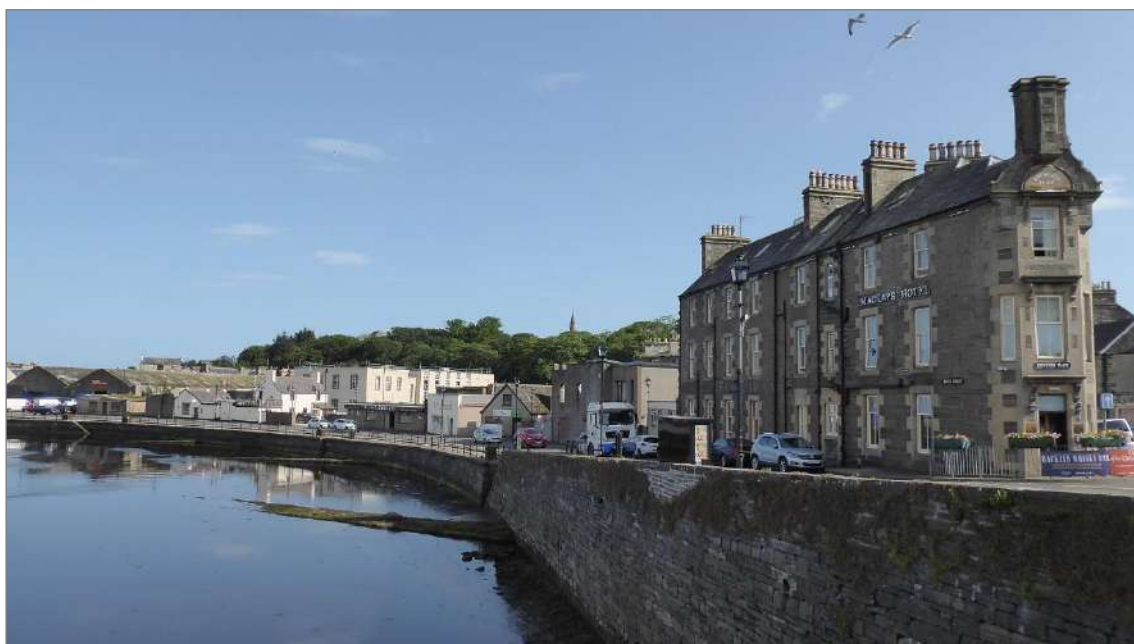
Figure 26: view of Lower Pulteneytown (River Street) from the Bridge of Wick. The majority of the street frontage has an inconsistent form and scale; however the street is anchored by the prominent Mackays Hotel cleverly fitted onto the narrow triangular site where River and Union Streets meet.
