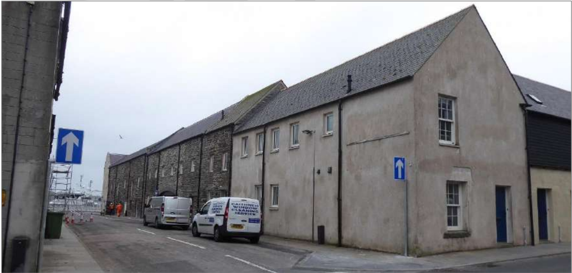
Figure 13: Parking and changes to traffic movement introduced as part of the regeneration of the eastern urban blocks either side of Telford Street: (top) open parking area created from former curing yards after loss of internal and street fronting buildings; parking area is highly visible; (centre) partly obscured parking within the block is a more sensitive approach although the finishes are still standardised they are less visible from the public realm; (below) to facilitate new uses Telford Street has been made one way with the standard blue signage standing out against the traditional finishes.
