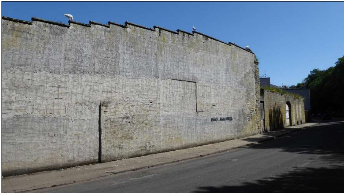
Figure 10: high masonry wall enclosing a plot on Union Street has a negative impact in terms of scale, materials, quality and monolithic style. It is unclear if original masonry fabric may survive below the rendered finish; earlier buildings on this site can be seen in historic images (e.g. fig 8)
