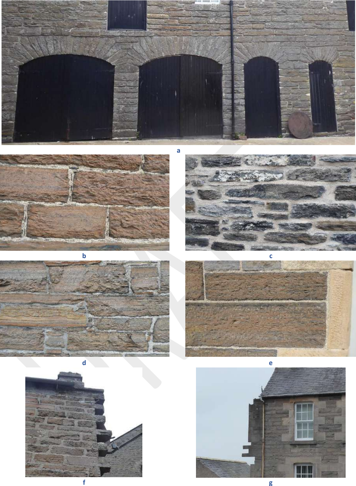
Figure 29: Masonry details: a: very fine examples of the segmental arches used in Pulteneytown particularly in the industrial buildings and to access internal yards, here at the Wick Heritage Centre; b: squared blocks of a warm brown Caithness stone with lime mortar and slate pinnings; c: walling recently repointed in lime on Saltoun Street warehouse, note the stones are more irregular in shape and darker grey in colour; d: a similar wall on a domestic property with irregular stones and courses, the gaps made up in smaller stacked stones; e: shaped Caithness stones on a Victorian building, cut to size, and used with sandstone dressings for openings; f and g: examples of masonry with projecting stones, known as ‘tusking stones’ or ‘tuskers’; left for bonding into the adjoining façade; image g showing the dressed window stones for the next property.
