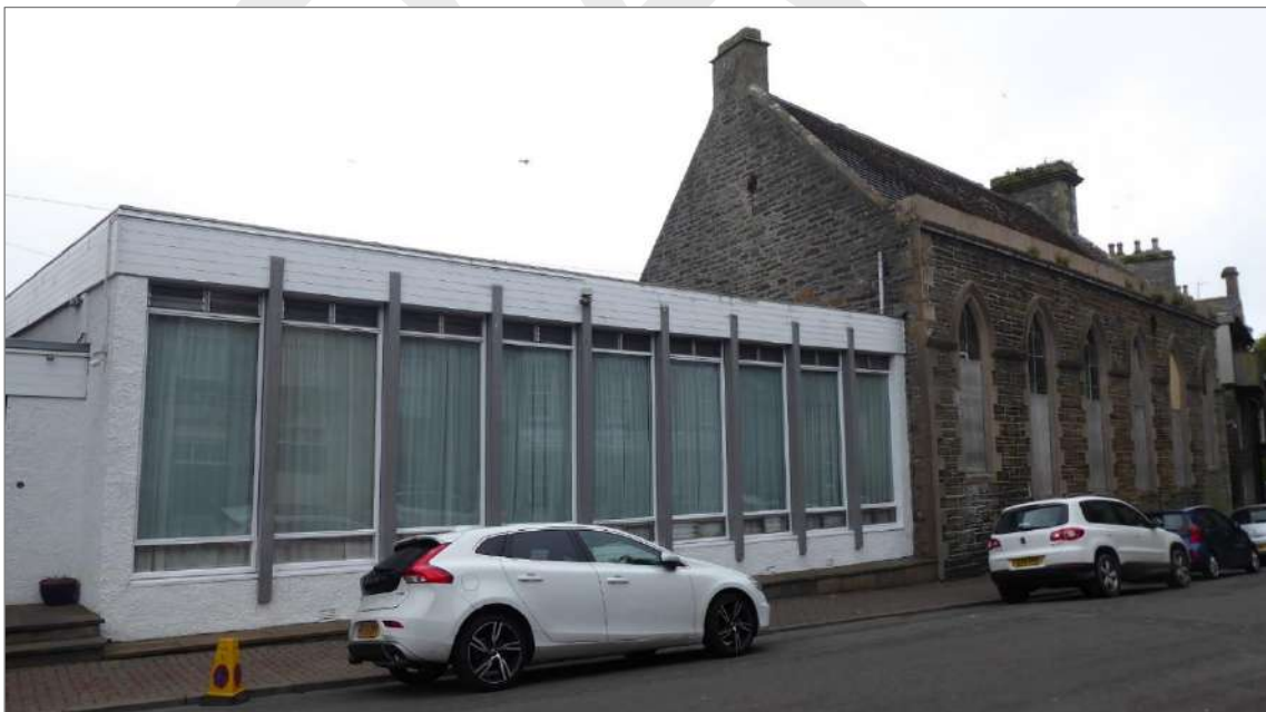
Figure 11: Inappropriate design: an example of a later 20 th century building design which is inappropriate to the character and appearance of the conservation area in terms of form (low horizontal emphasis and flat roof), materials and colour, the bright white is in stark contrast to the adjacent stonework and draws further attention to the building. Buildings such as this may offer opportunities for redevelopment or enhancement through planning management.
