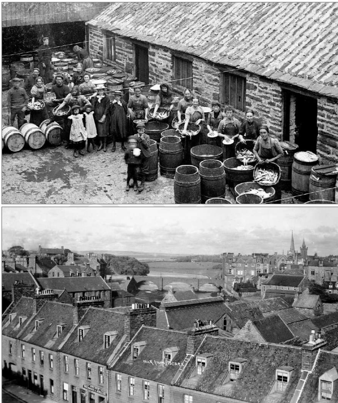
Figure 31: (top) George Cormack’s yard in Lower Pulteneytown in 1900s with pantiles on the roof of the single storey building and what looks to be a Caithness slate easing course at the eaves; a rough cobble stone finish to the yard; (below) Historic view over the roofs in Union Street illustrating the predominance of slate roofing but with other finishes including pantile on some industrial buildings. © The Wick Society - The Johnston Photographic Collection
