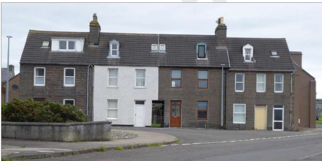
Figure 45: (top) pre-1839 properties forming the eastern row of Smith Terrace and similar original houses on Vansittart Street (below) all part of Telford’s plan and having been feued by George Burn; part of Lot 1 on Vansittart Street was constructed by 1813, thought to be Nos. 5 & 6 on the left of the pend. Both rows out with the conservation area.
