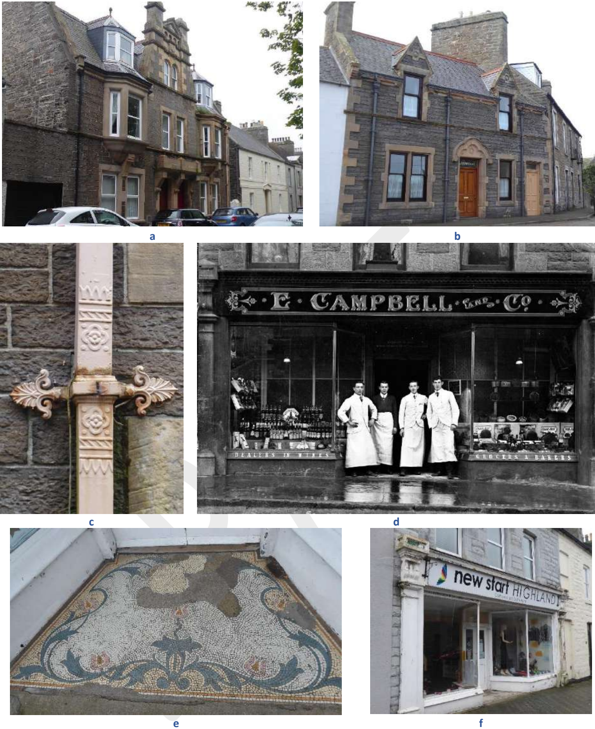
Figure 35: Victorian buildings: a: Nos. 15 and 16 Sinclair Street are elaborate Victorian style houses which dwarf their Georgian neighbours and exhibit much of the change in design and material use by the end of the 19 th century; b: a more modest Edwardian house on Breadalbane Terrace built in 1911 with again more intricate stonework and decorative cast iron rainwater goods; c: decorative square downpipes and acanthus holding brackets at 15 and 16 Sinclair Street; d-f: just out with the conservation area, a late Victorian shopfront survives with a traditional terracotta mosaic entrance platt, originally E. Campbell & Co. Grocers. (Historic image © The Wick Society - The Johnston Photographic Collection).
