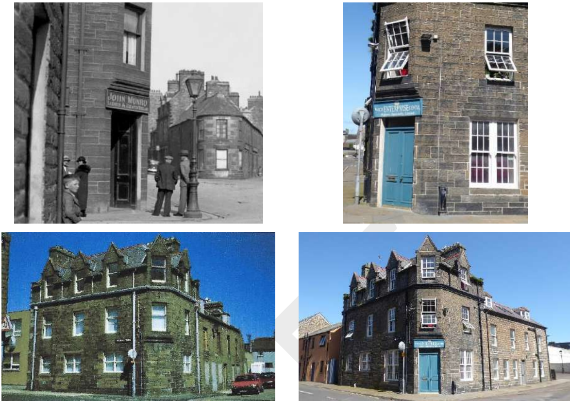
Figure 5: illustrating the importance of following window guidance fully. On the left an image from the 1930s showing likely original window and door design with below the building in 2000 with the same window pattern (door built up). The building in 2019 (right) has new replacement windows which have not replicated historic evidence and the opening form does not comply with current guidance that window opening methods should not disrupt the elevation. 6 over 6 pane windows may be the correct pattern for some earlier buildings in the conservation area, but the date of this property in the late 19 th century would suggest it is less likely and such windows would rarely combine ‘horns’ in the original design. The reinstatement of the door is however a positive enhancement.
