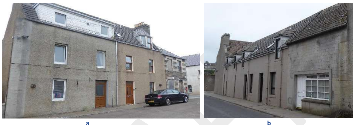
Figure 37: modern cement finishes applied to traditional buildings; also note on a: the large box dormer which has a negative impact on the building frontage and roofscape; and b: again shows the presence of concrete tiles, here next to a restored traditional Caithness slate on the roof to the right.
