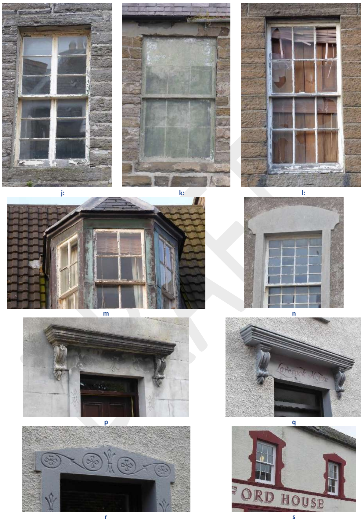
Figure 34: Window and doors: j: original lying pane windows at 2 Union Street; k: blind window on Smith Terrace; l & m: typical 6 over 6 Georgian window with internal shutters at 17 Breadalbane Crescent, with 4 over 4 pane dormer window to attic; n: distinctive multiple pane window on former Wick Free Church on Malcolm Street; p-r: examples of incised detail on door surrounds, console brackets and moulded lintels in Argyle Square; s: unusual window margins to Telford House in Lower Pulteneytown.
