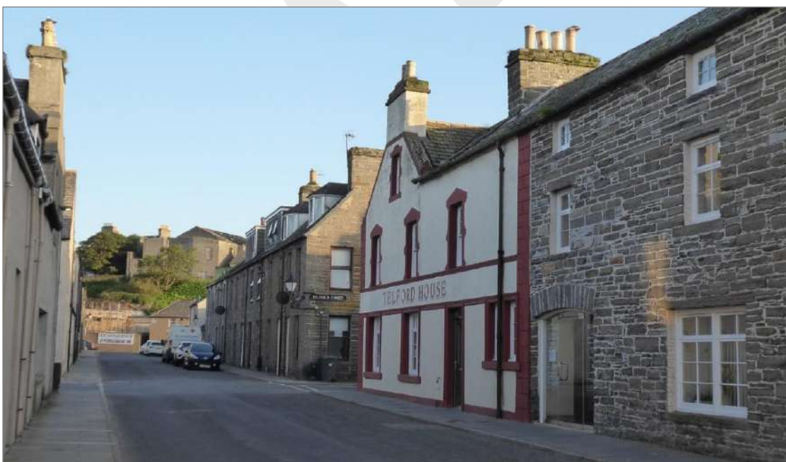
Figure 15: the consistent eaves line on Williamson Street (west side). Note how the 3-storey warehouse on the right maintains the eaves line of the neighbouring 2-storey Telford House.
