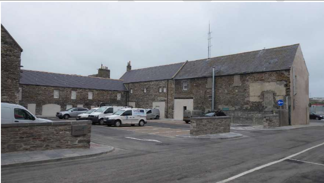
Figure 10: Two lots on north side of Telford Street which address Harbour Quay were repaired c.2012 as part of the Beatrice Offshore grant / investment. The buildings are still awaiting a new use. The former herring curing yard was a scrap metal yard in 2008 (top, © Google Maps); the Telford Street fronting buildings appear to have been demolished sometime before the repair work, which consolidated existing buildings (below 2019). No structures remain from the original buildings which divided the two lots. The site offers further potential for street frontage infill which would also obscure the open car parking site from view.
