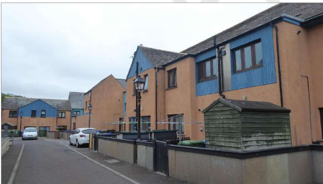
Figure 10: recent redevelopment on Saltoun Street has reduced the hard frontage of the block and set housing back from the street line with small front yards and parking.
