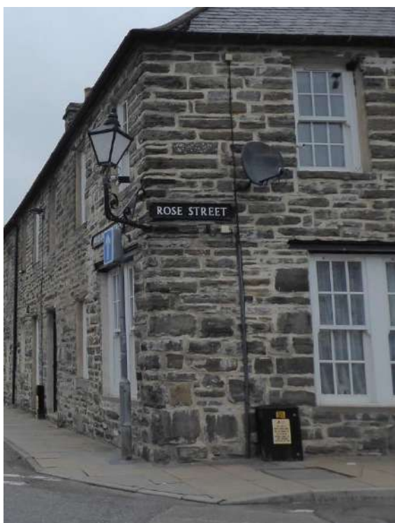
Mixed and cluttered street furniture: enhancement gained by using a traditional lantern and street sign is offset by cabling, satellite dish position and standard one-way road sign. Note the dropped kerb using Caithness flagstone.
