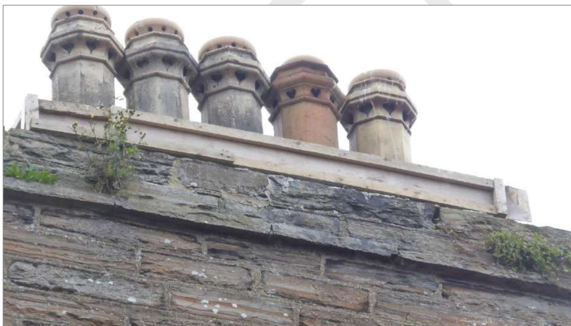
Figure 33: a typical Pulteneytown chimney with a thin flagstone slab forming a projecting tabling course detail before a further one or two courses of stone form the cope. Here with more elaborate hexagonal buff coloured chimney pots.
