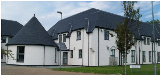
Elgin Residence (credit: Archive Centre webpage)
